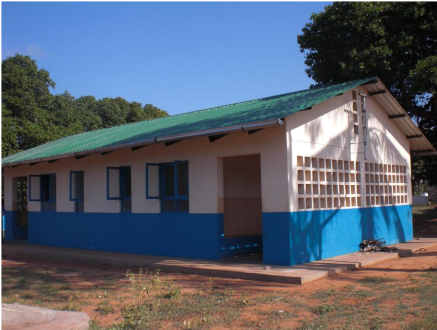
Figure 5.2. MWH in Mucojo health facility
