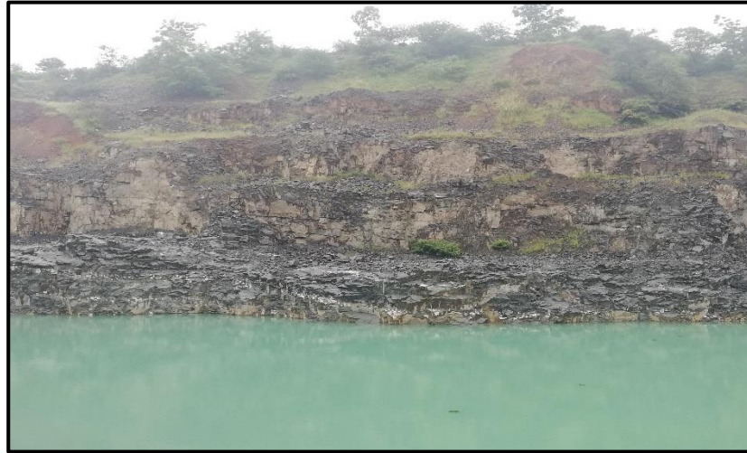
Figure 4. 3: Slope C benches layout and evidence of water accumulated at the pit floor.
