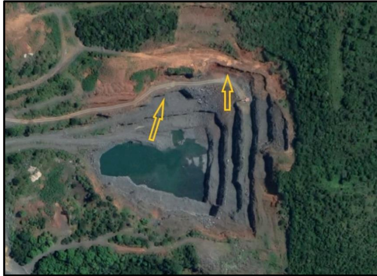
Figure 3.2: Areas in Section A of the open pit mine with wider benches.
