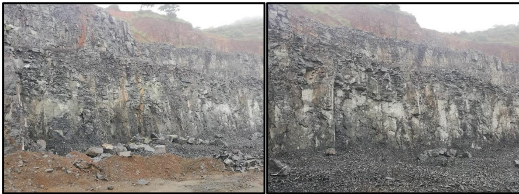
Figure 4.1: Slope A benches and dominant discontinuities on the slope.
