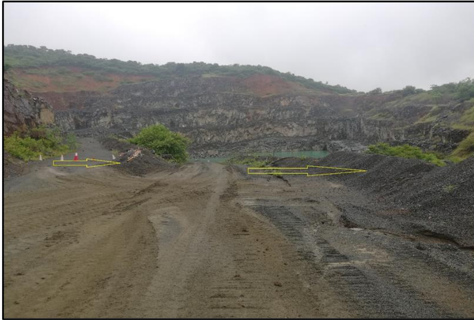
Figure 4.4: catchment berms of the open pit indicated by yellow arrows.
