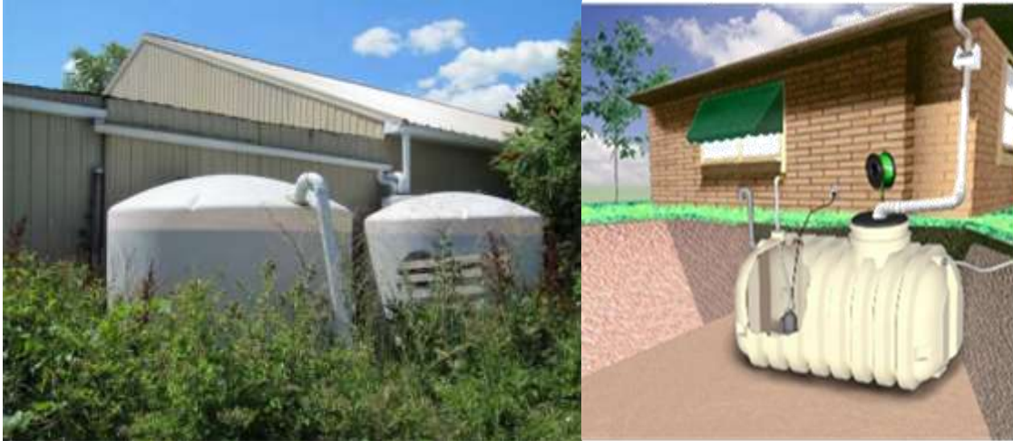
Figure 9: Photograph of above-ground polyethylene water tanks and diagram of underground rainwater tank. Source: Islam et al. (2013) and Scarfiello (2015)
