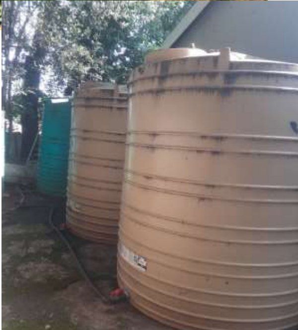
Figure 31: Jojo tanks used for wastewater recycling and for storing water. Source: Author
