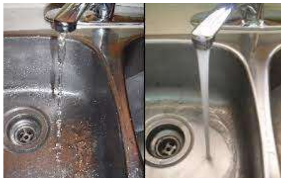
Figure 7: Difference in water flow between a non-aerated tap and an aerated tap. Source: Visser (2021)
