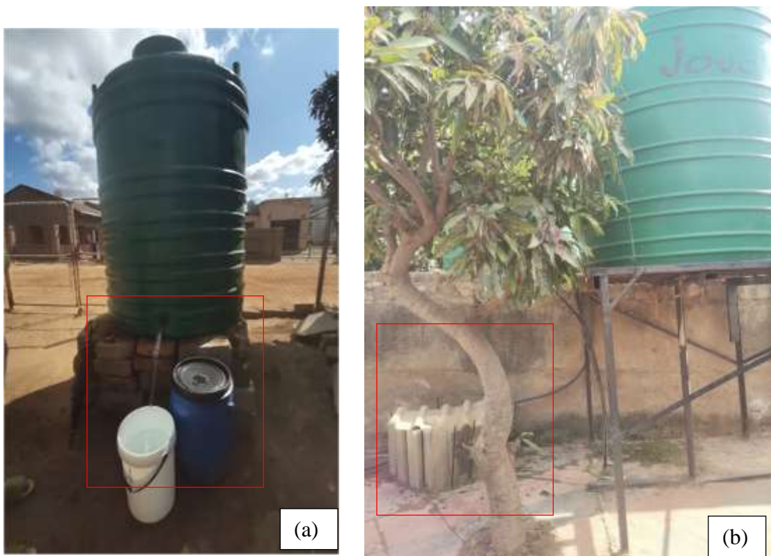
Figure 27: (a) Photograph of clean water from hand dug wells that are connected to jojo tank; (b) Photograph of a covered homedug well that is used as a water supply in a household in Hammanskraal. Source: Author
