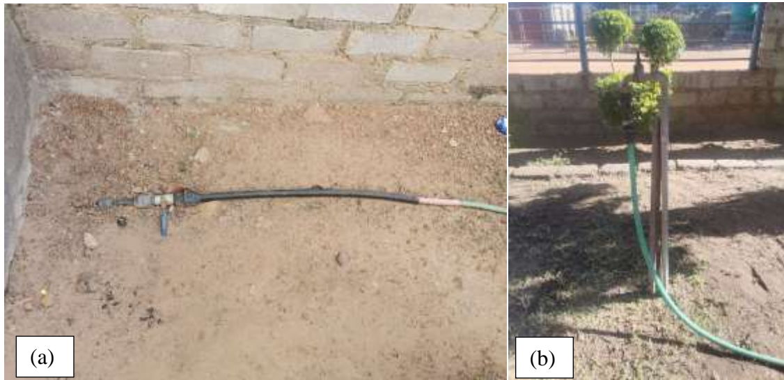
Figure 24: Available pipelines and taps available as infrastructural resources to supply water services to the households in Hammanskraal. Source: Author
