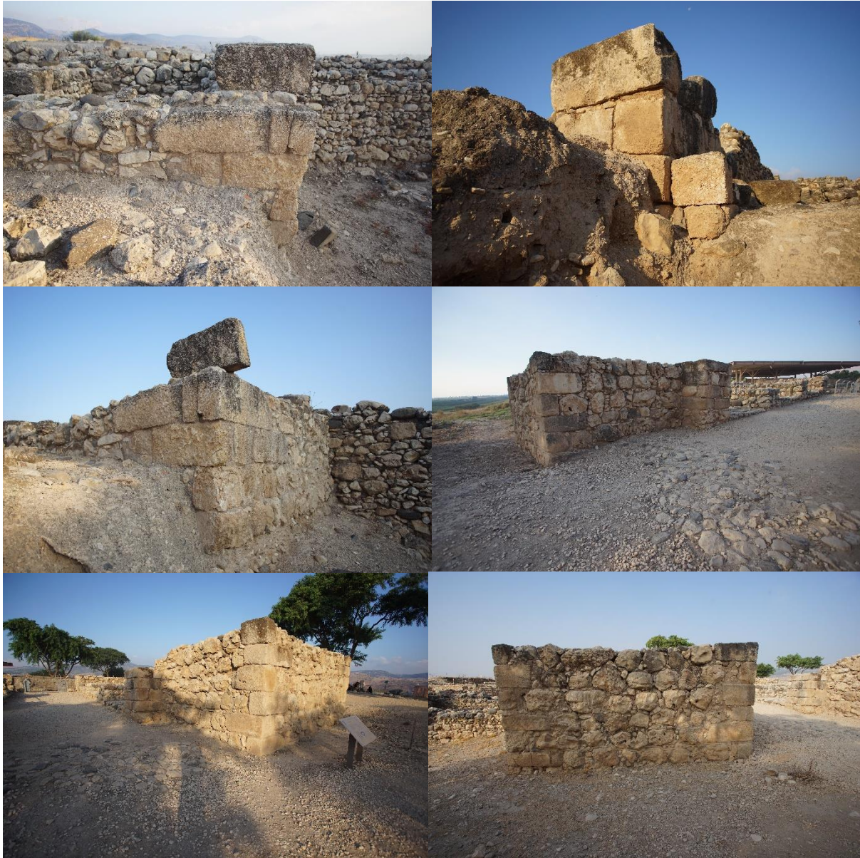
Figure 7.5: Examples of Ashlar masonry at Tel Hazor (Photos: MC/The Selz Foundation Hazor Excavations in Memory of Yigael Yadin)
