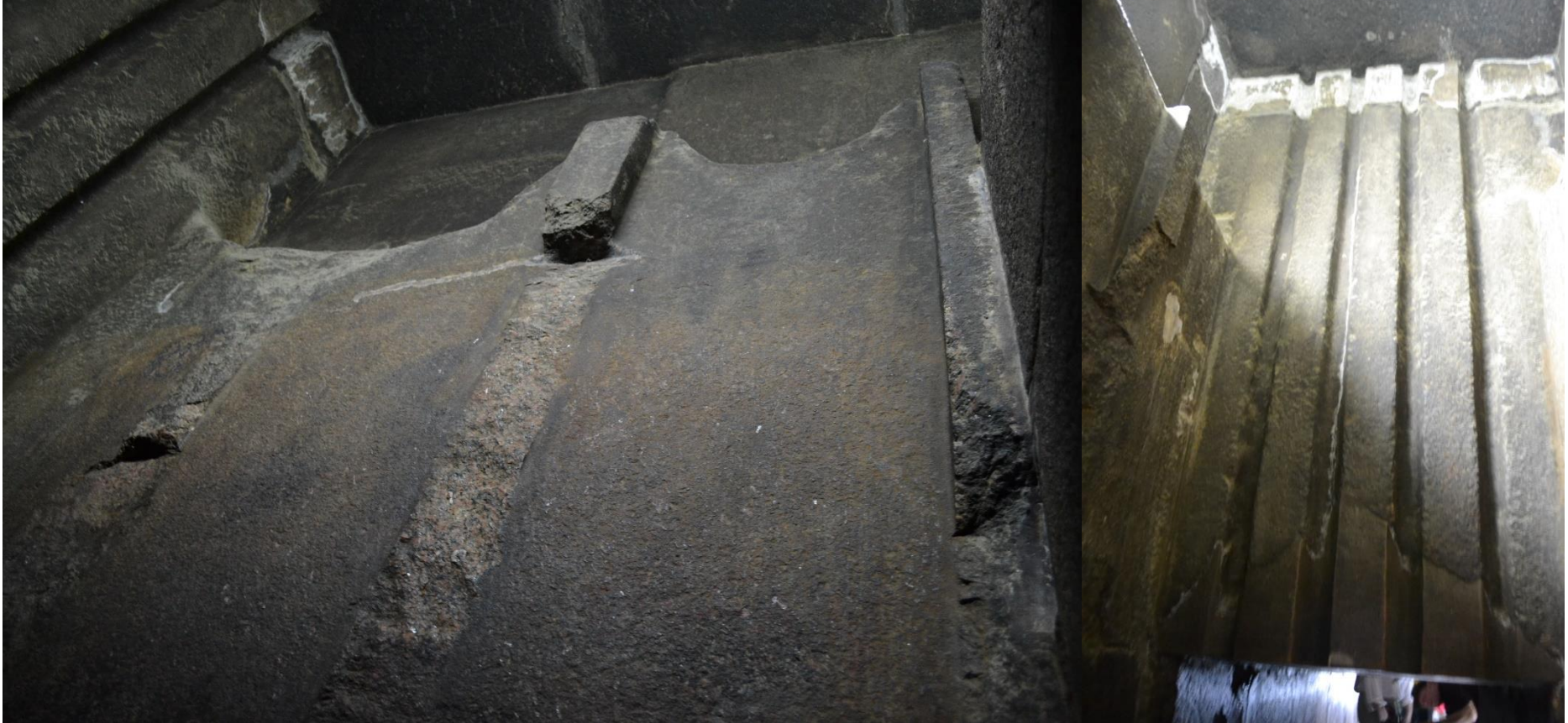
Figure 2.10: Slots for plugs and portcullises at the entrance to the burial chamber in the Great Pyramid (Photos: NB Hoffmann September 2022)
