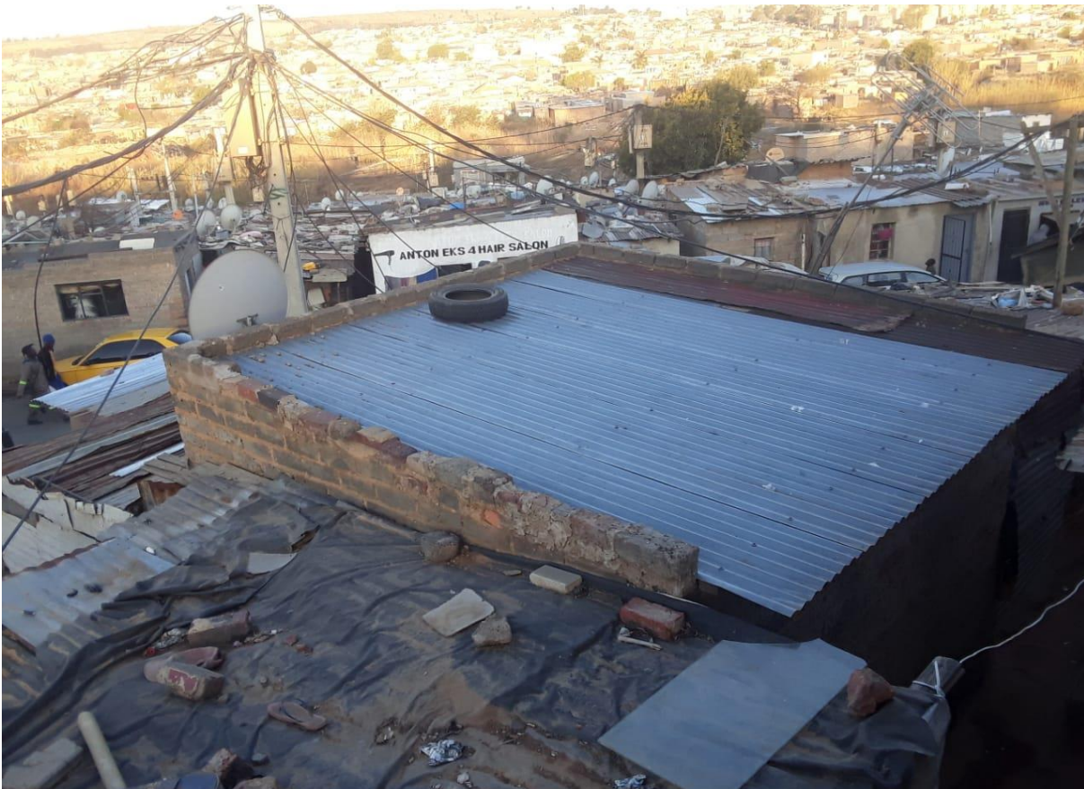
Image 4-2: Some of the houses with metallic sheet roofing
