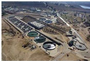
Northern wastewater treatment plant (WWTP)
