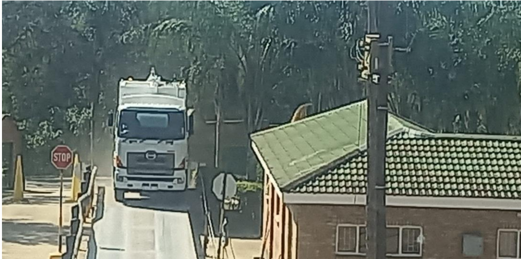
Photograph 3.1: Tzaneen Landfill Site weighbridge where quantity of tonnes for solid waste are calculated.
