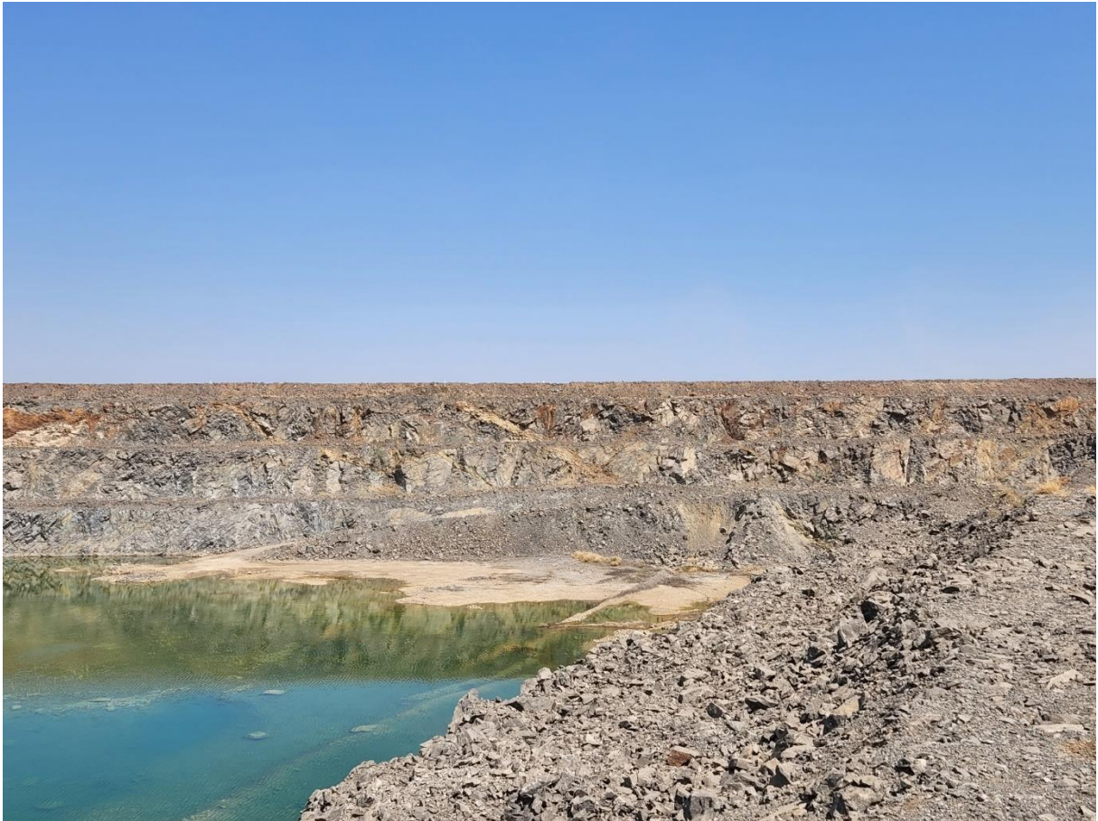
FIGURE 4.6: CURRENT GROUNDWATER LEVEL AT THE PIT (29 AUGUST 2022).
