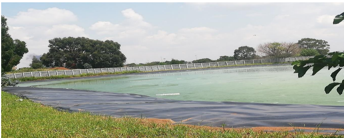
Figure 4.3: Leachate dam at Rietfontein Landfill Site (13 February 2020)
