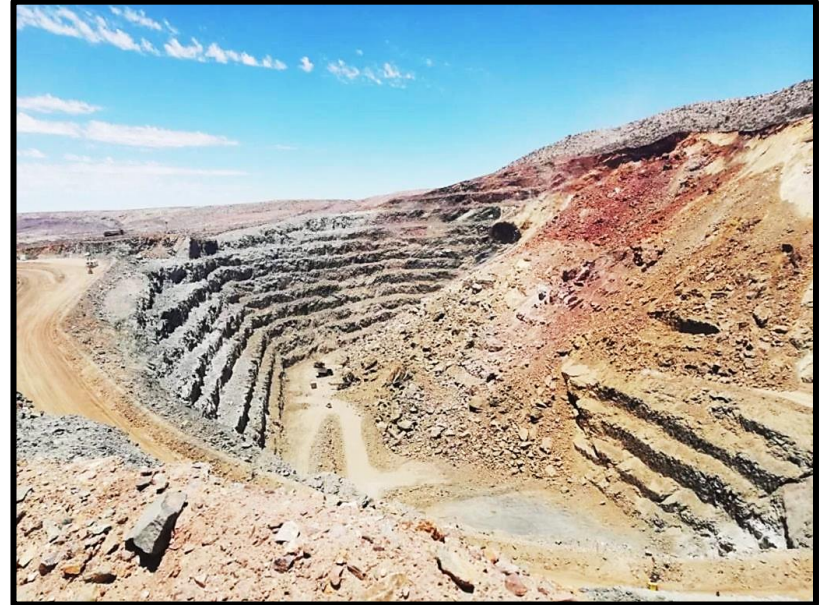
Real operation with failed slope
