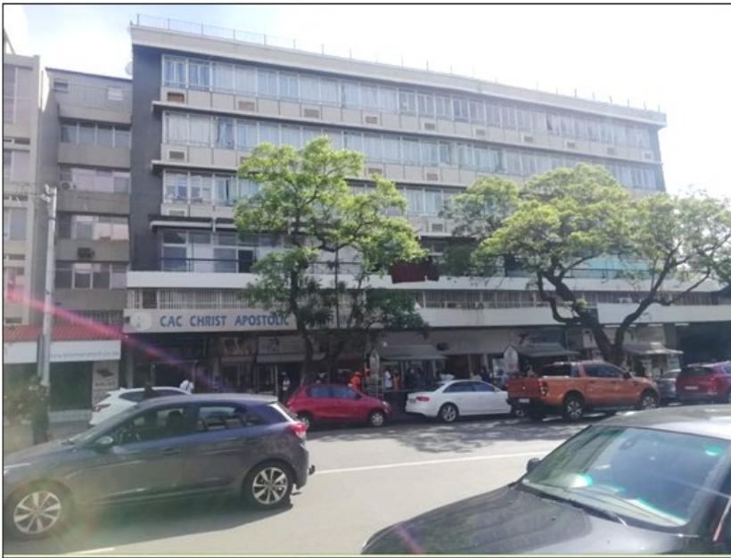
Figure 5.1: The Sunnyfair building on Robert Sobukwe Street, Tshwane (Captured by the researcher, 10 November 2021)
