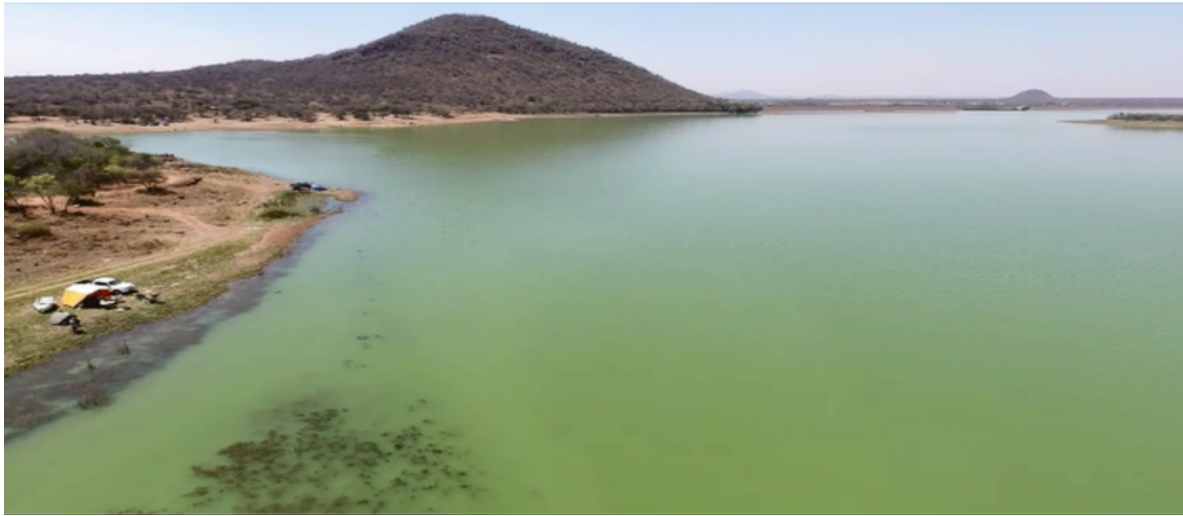
Figure 1.2: The Vaalkop Dam
