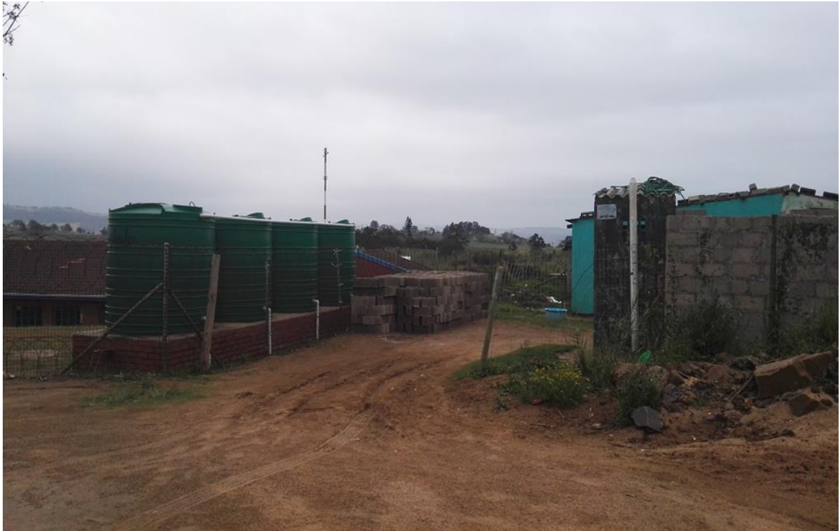
Figure 4.16. Tanks where households store harvested rainwater in Etete. Source: Researcher (2021).
