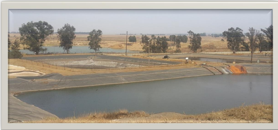
Figure 3.8 HPDE lined leachate dams where leachate is stored and treated to reduce the toxicity levels of the leachate.
