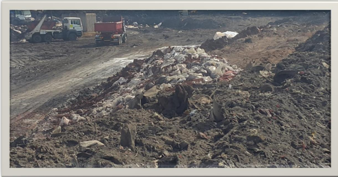
Figure 3.7: Operational cell at waste disposal site where trucks are disposing waste
