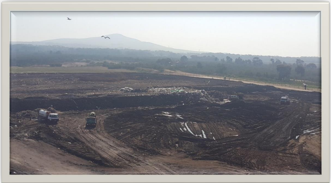
Figure 3.11 An operational cell and the working face of the site
