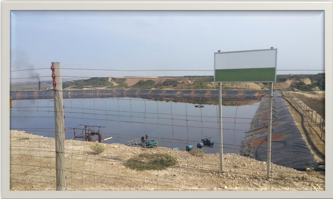
Figure 3.10: A leachate dam at a site
