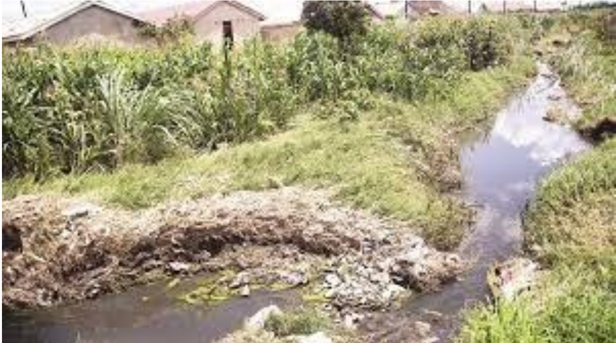
Figure 5.6: Conditions of wetlands in Gweru City (Source: Fieldwork)
