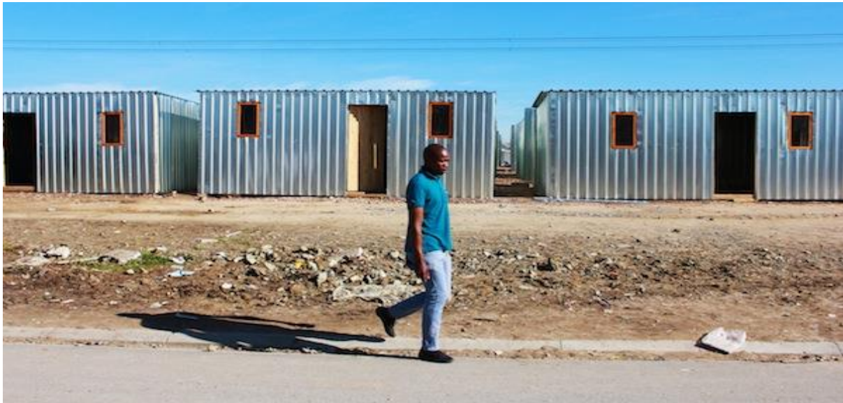
Figure2: Restructuring the shacks to avoid spread of fire.
