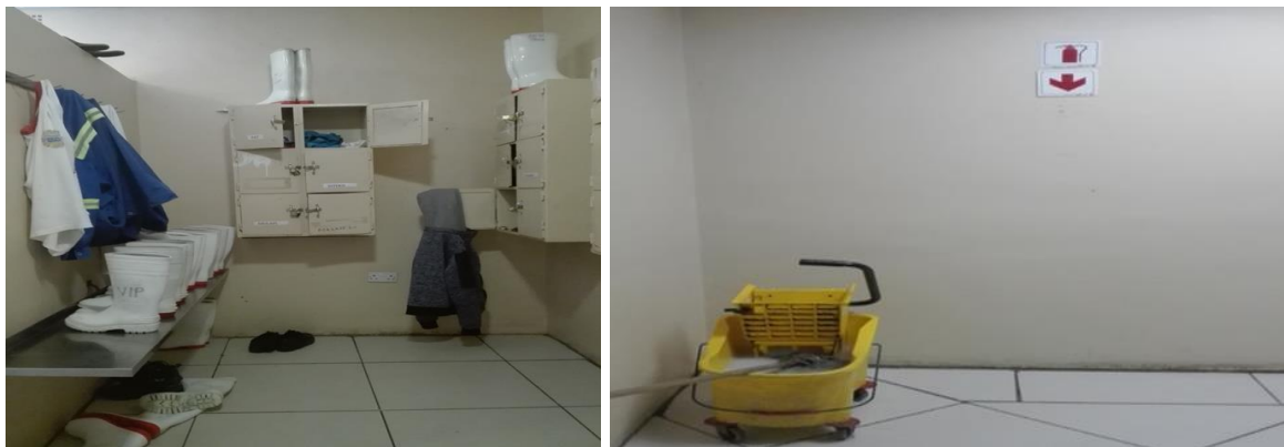
Figure 3: No labelling and floor markings
