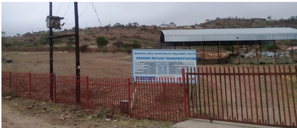
Figure 4.13: Dzanani Transfer Station
