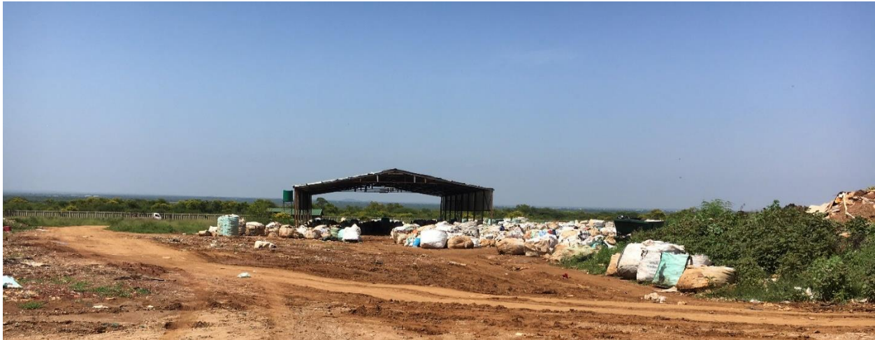
Figure 4.16: Recycling facility within Makhado Landfill Site
