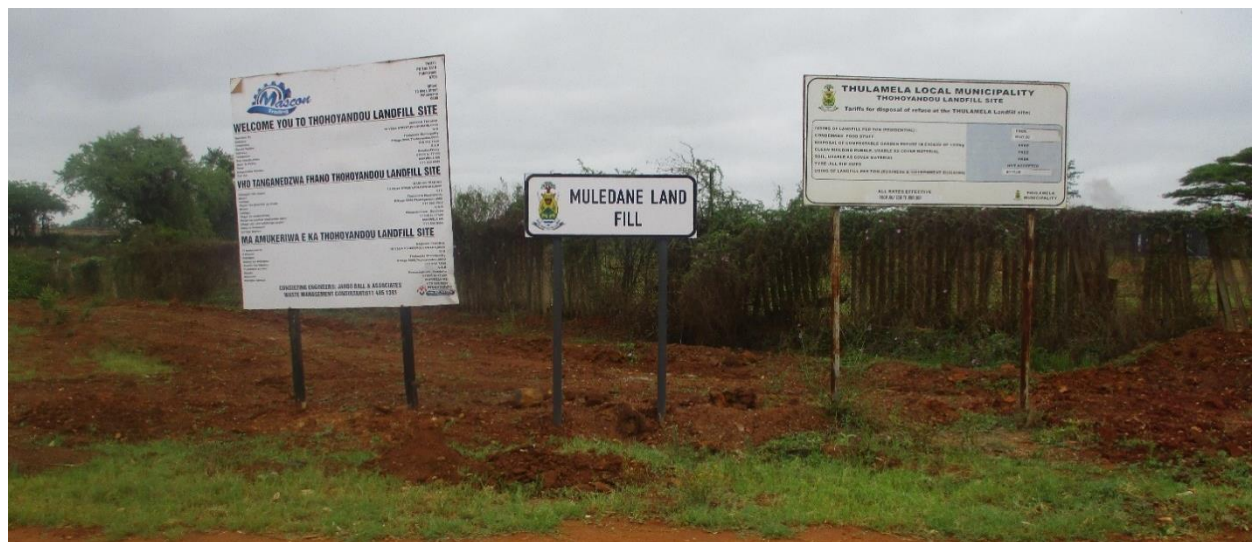
Figure 4.18: Notice Boards at Thulamela Landfill Site entrance
