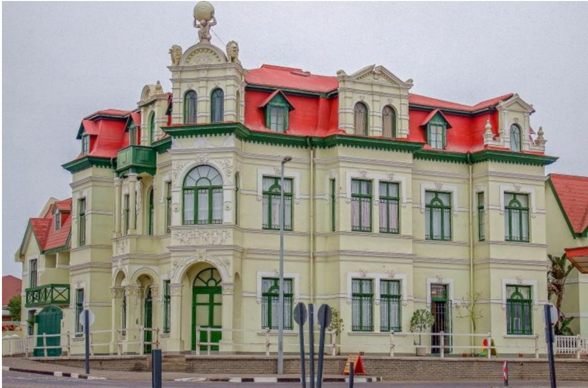
Figure 4.4: Hohenzorllern Building, Neo-Baroque style. Source: Author (May 2021).
