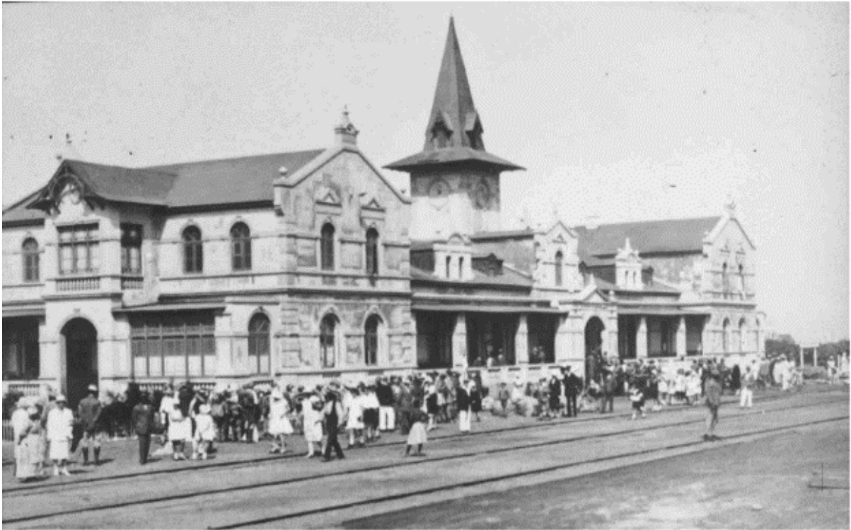
Figure 4.2: Railway Station Building, Rundbogenstil style merged with Renaissance features. Source: Decker (2020).
