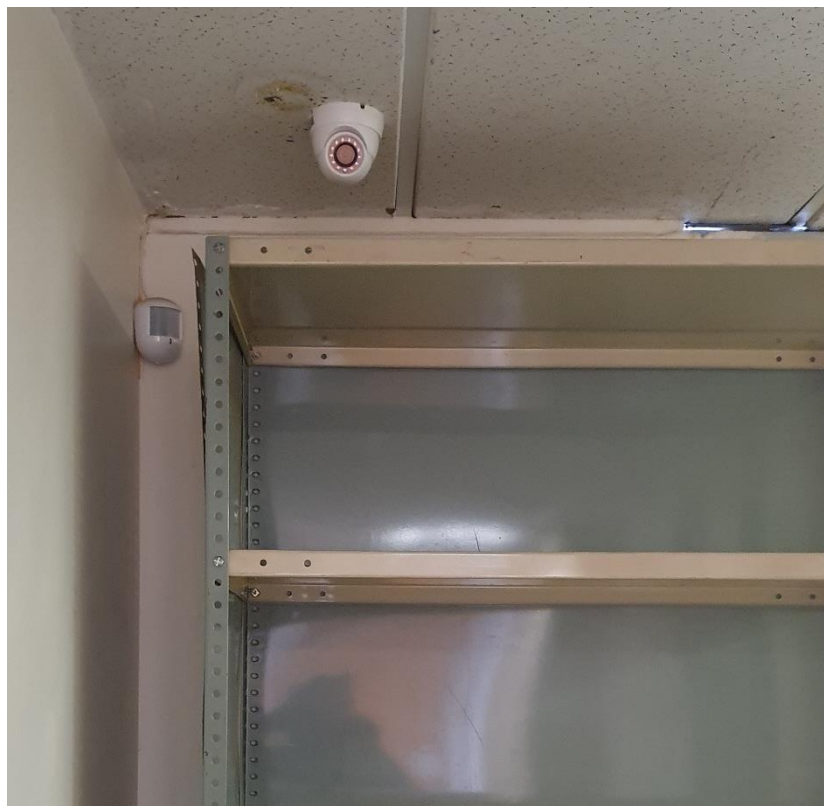
Figure 4-41: Surveillance camera (Photographer: Researcher 2020)
