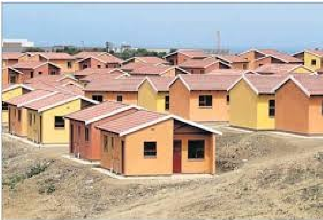
Figure 5.4: South Africa's RDP houses
