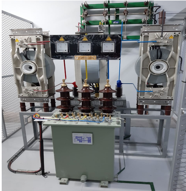
Figure 3.12: Coupling cell
