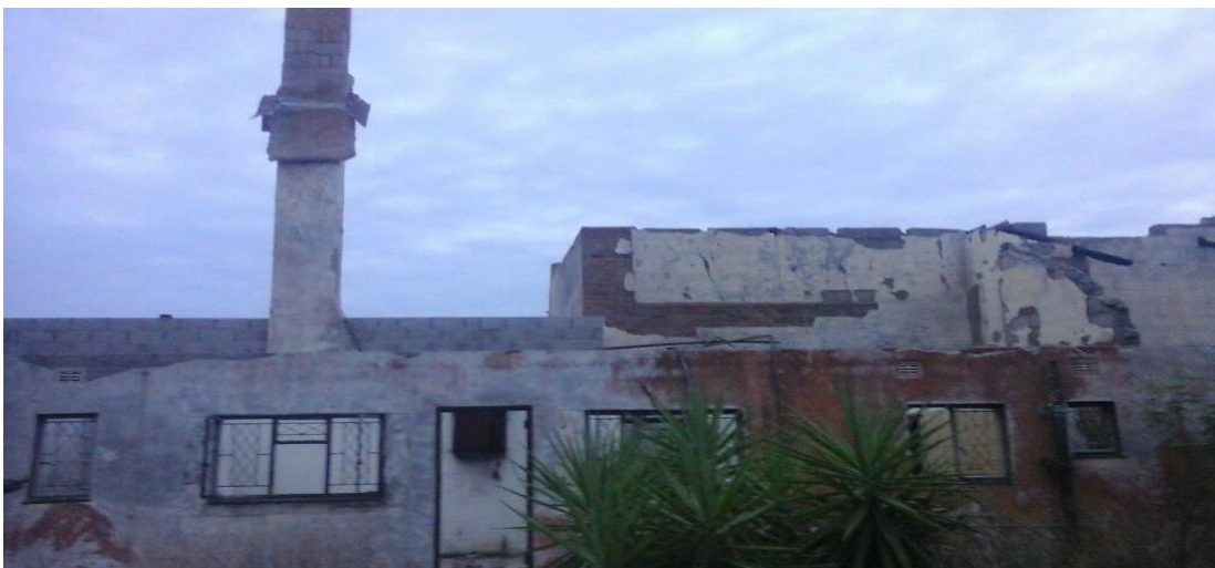
Fig 4.9 Showing Dingwall Game lodge that was destroyed by fire in 2015
