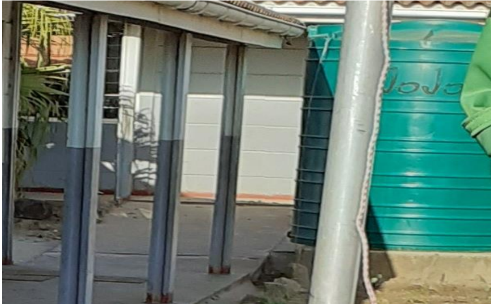
Photo 4.4: A JoJo tank for harvesting rainwater at Luge primary
