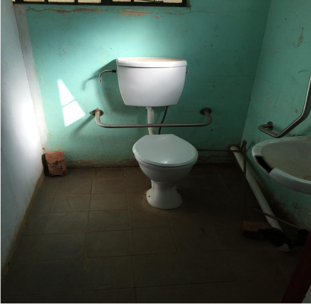
Figure 5: Koti Primary's paraplegic toilets
