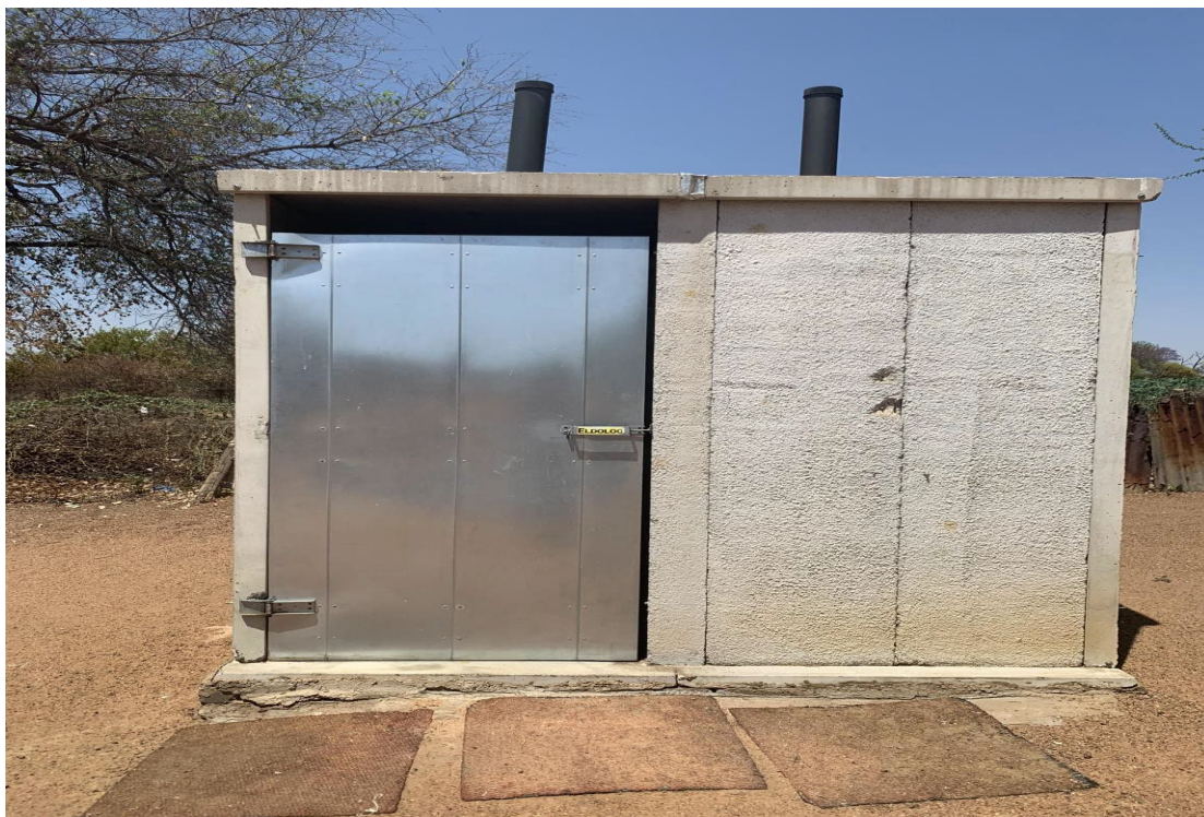
Picture 3: Urine Diversion System: residents in Winterveld had benefitted from the government sanitation programme
