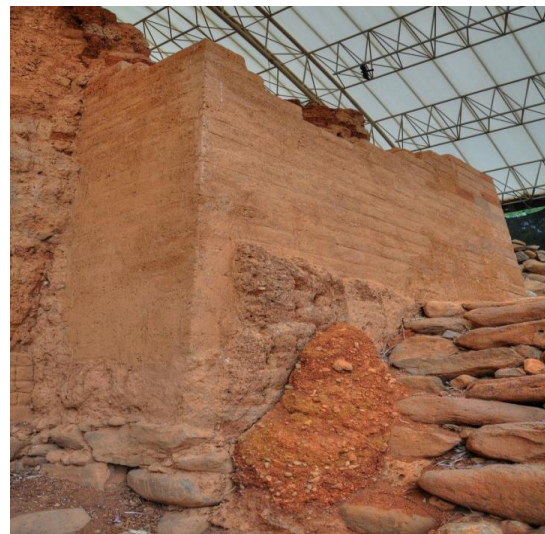
4. Mudbrick wall plastered
