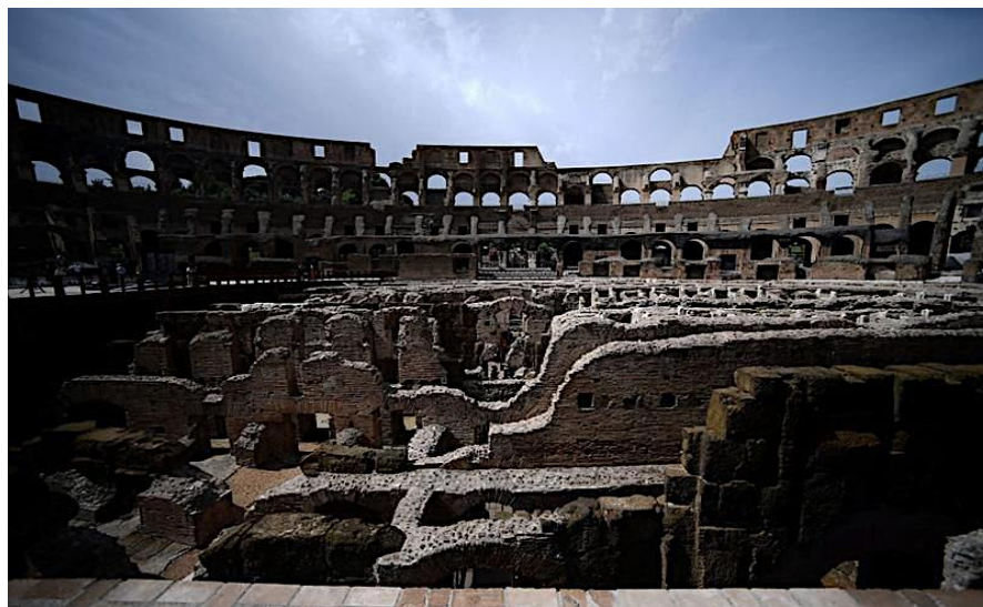
Figure 4.24: Showing the hypogeum , the interlinked underground tunnels underneath the arena.
