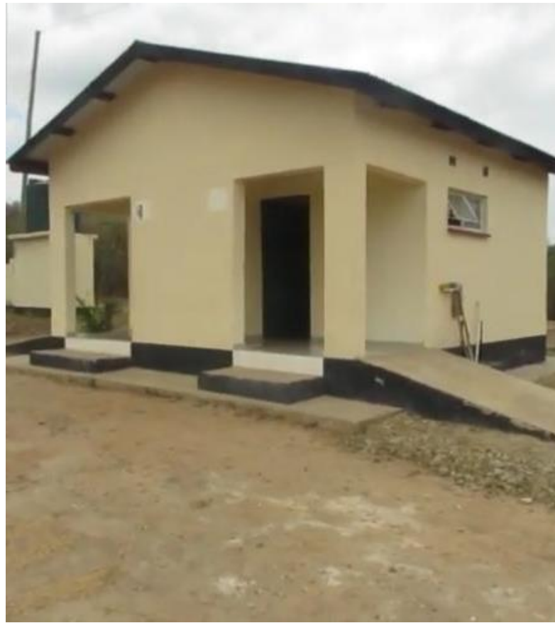
Figure 4.17: A toilet structure at Chinyunyu thermal springs
