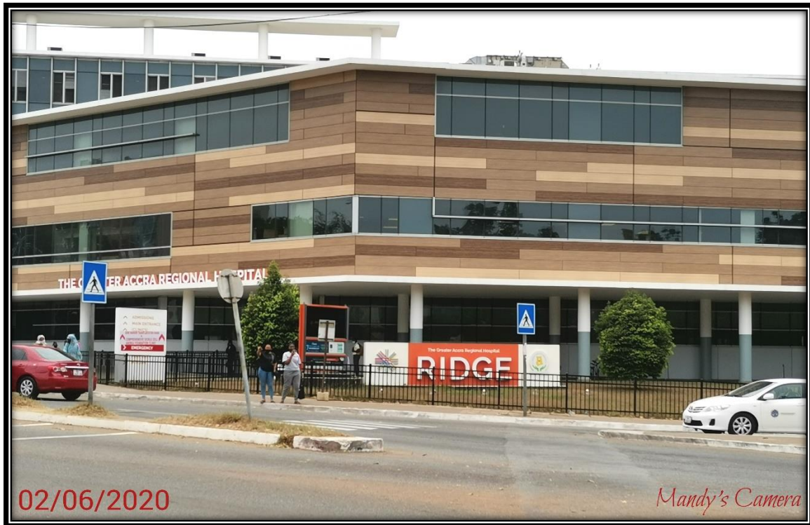
Figure 5. 6: The Greater Accra Regional Hospital (Ridge Regional Hospital) Source: Field Data 2020
