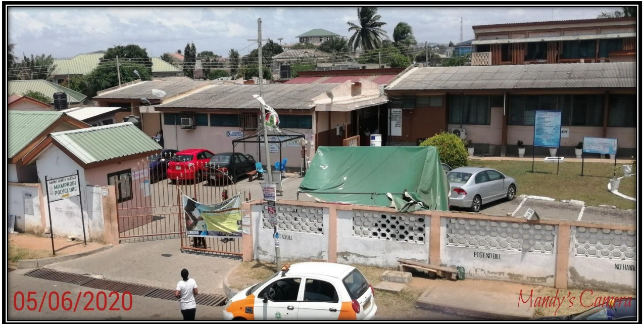
Figure 5. 8: Mamprobi PolyClinic Source: Field Data 2020.
