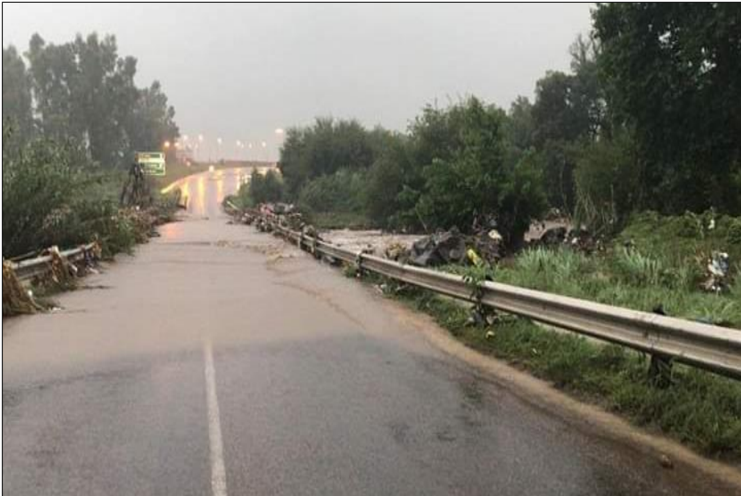
Figure G.1: Flooded road in Centurion
