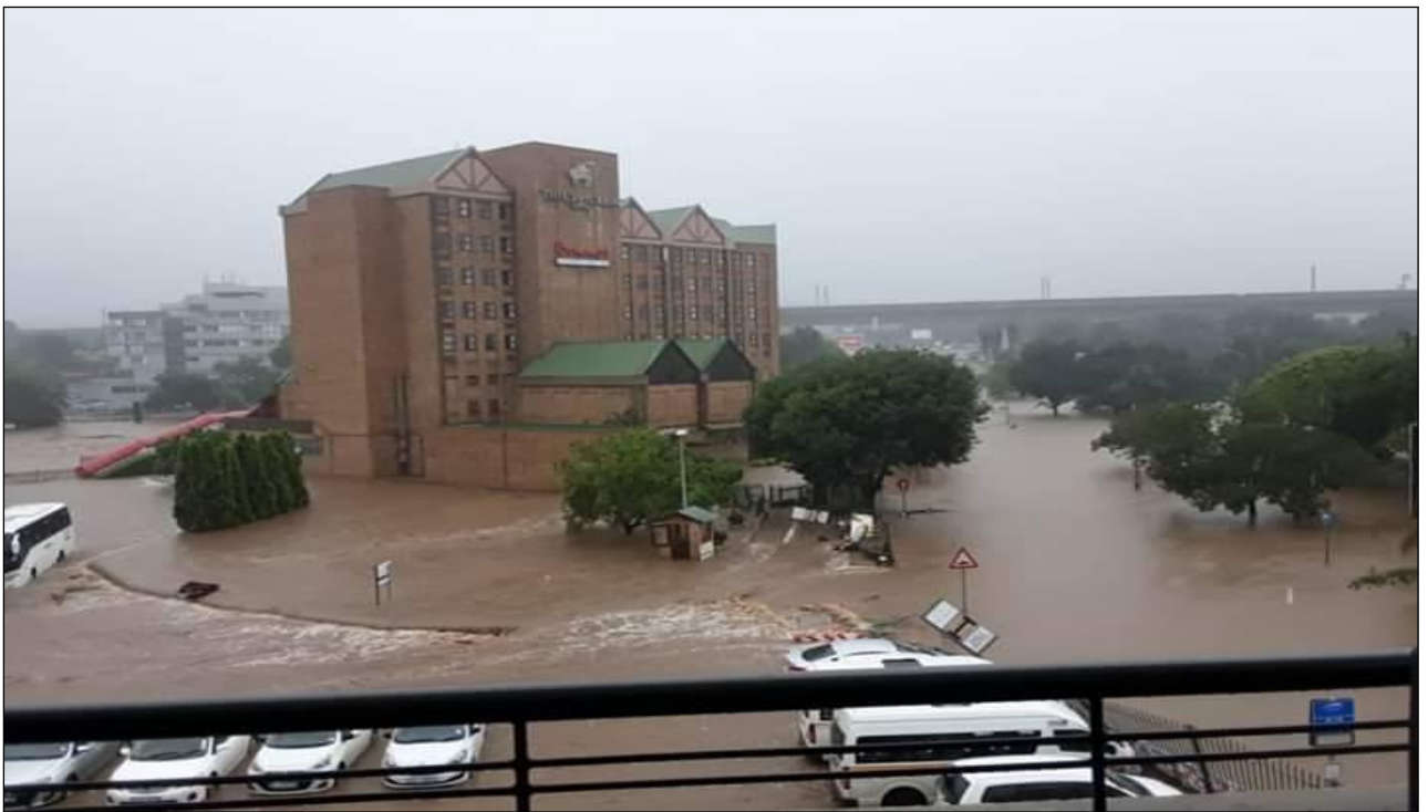
Figure 7.3: Centurion CBD flooded
