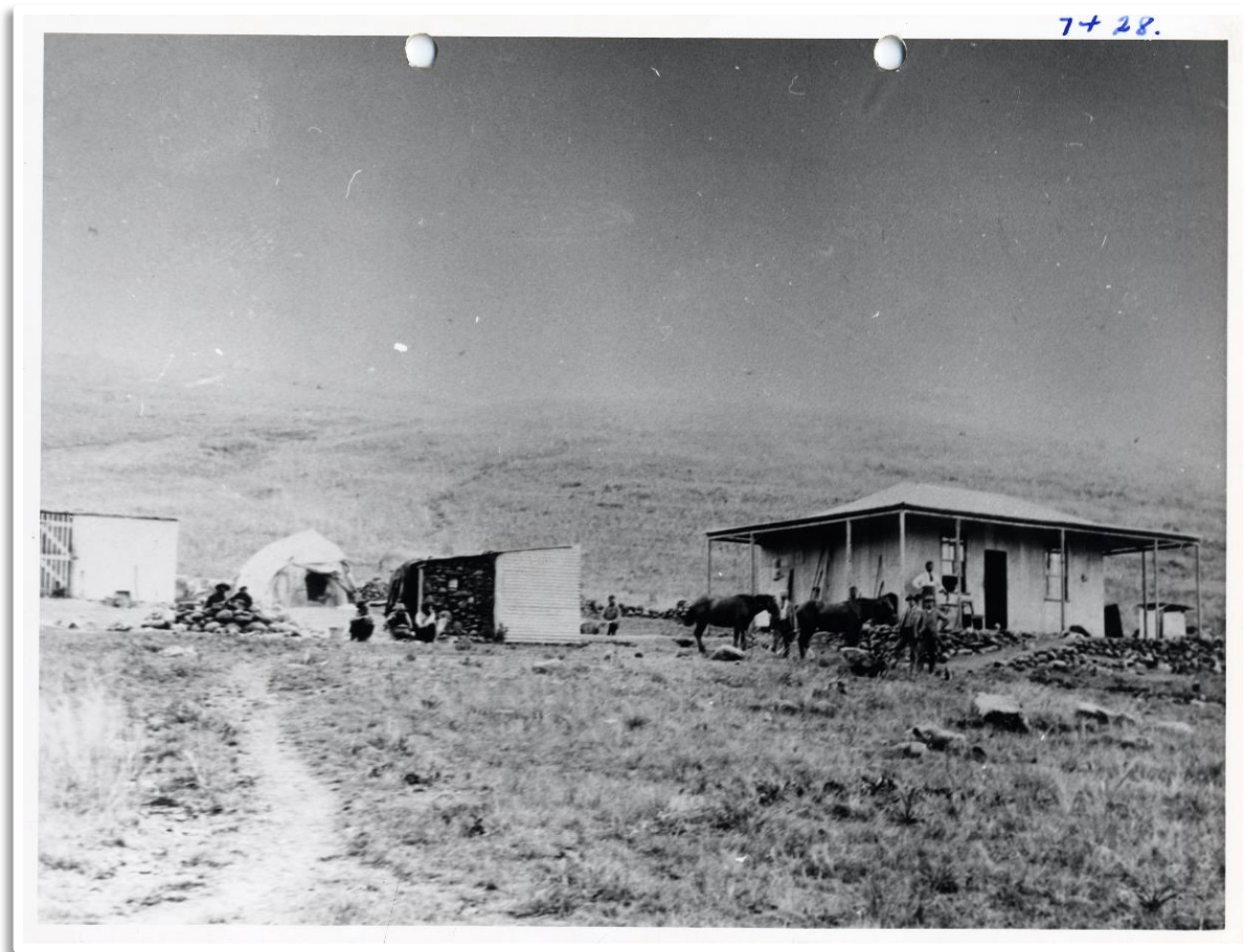
Figure 8 Prefabricated corrugated-iron cottage and outbuildings in the camp at Pampoenspruit, KM 215. Photo: National Archives Repository TAB7428.
