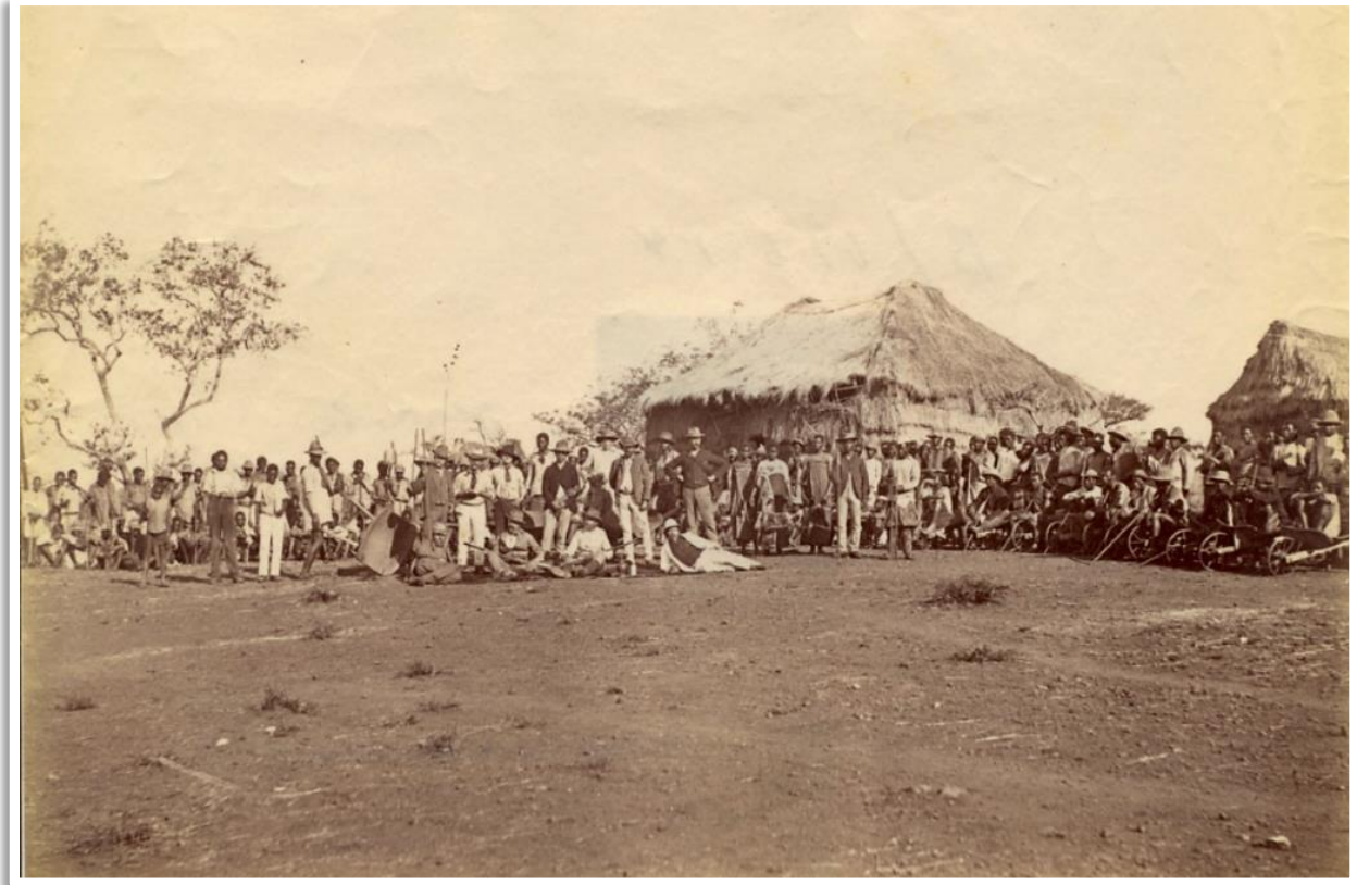
Figure 5 European and African construction workers pose at Reid's camp, 1892. Photo: Het Zuid-Afrikahuis Map71-17a 1257.
