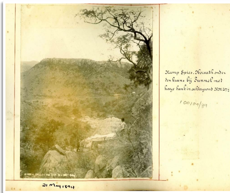
Figure 51 “Camp Spies. Horvath underneath the cliff, at the Tunnel, with high embankment in the background KM 207.5”. Waterval-Boven May 1894. Photo: Transnet Heritage Library and Archives 100109/39.
