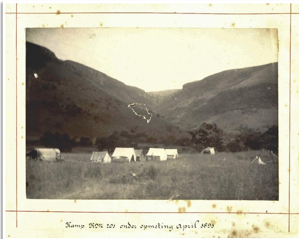
Figure 4 Surveyor's tented camp at KM 201, April 1891, Caney, W & Co. Photo: Transnet Heritage Library and Archives 100109/2
