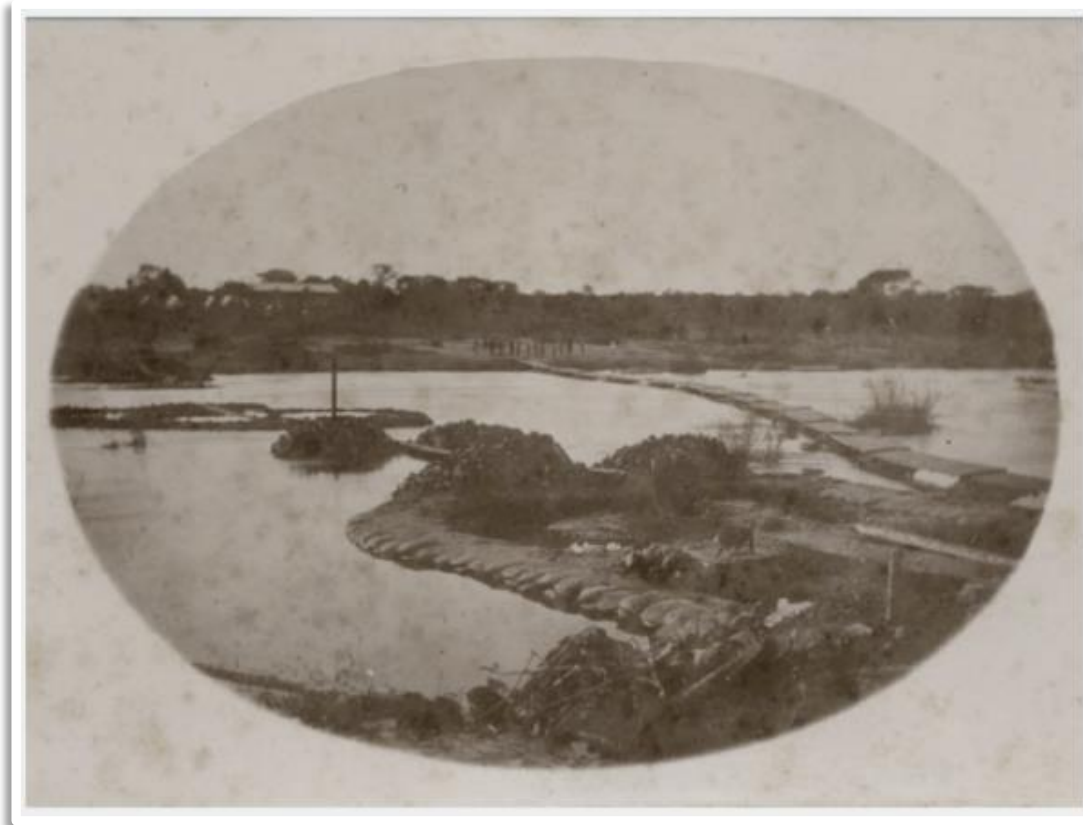
Figure 23 Early days of the construction of the Komati River Bridge with the footbridge to the right, 1890. Camp on the northern bank of the river, top left in the photograph. Photo: Het Zuid-Afrikahuis Map69-21 1202.
