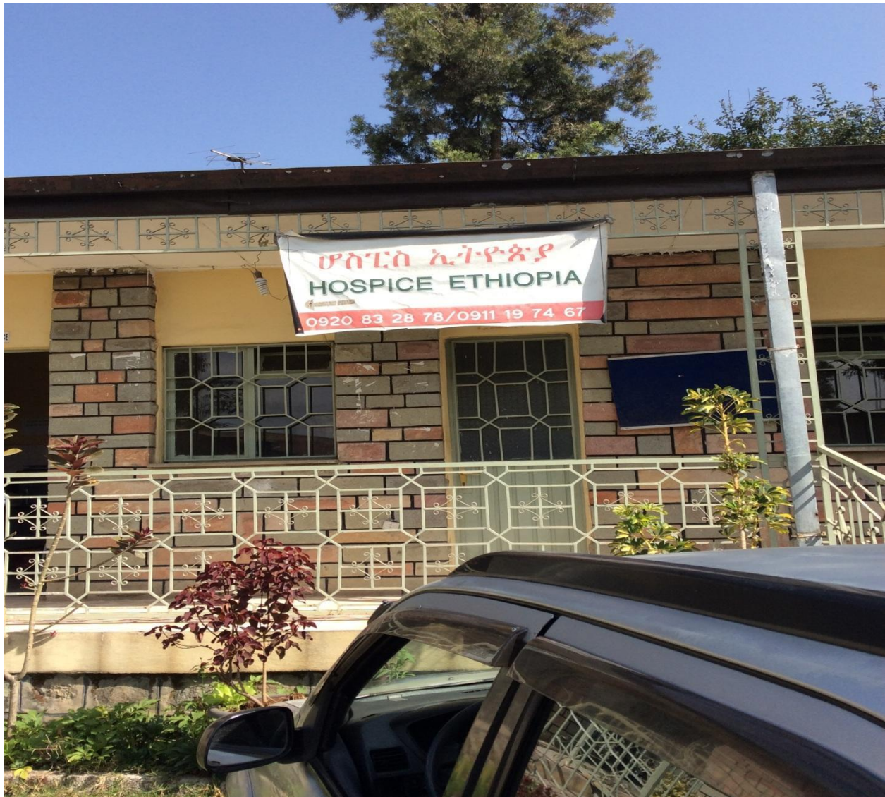
Figure 4.2 shows partial view of Hospice Ethiopia, Addis Ababa,kotebe kara yeka
