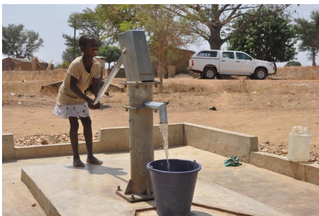
Figure 6.10: Functional borehole, Nhyiaeso
