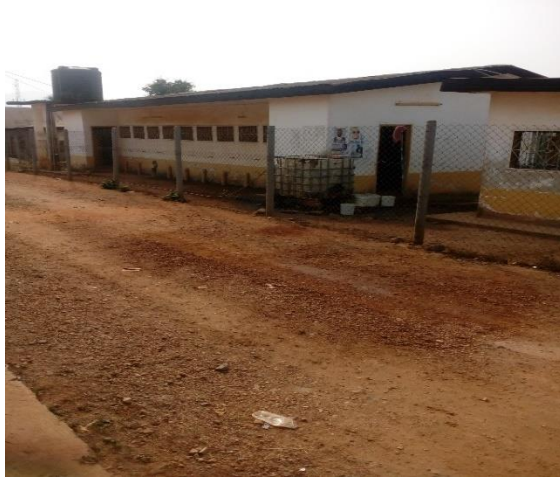
Figure 6.8: Functional toilet facility, Bidiem
