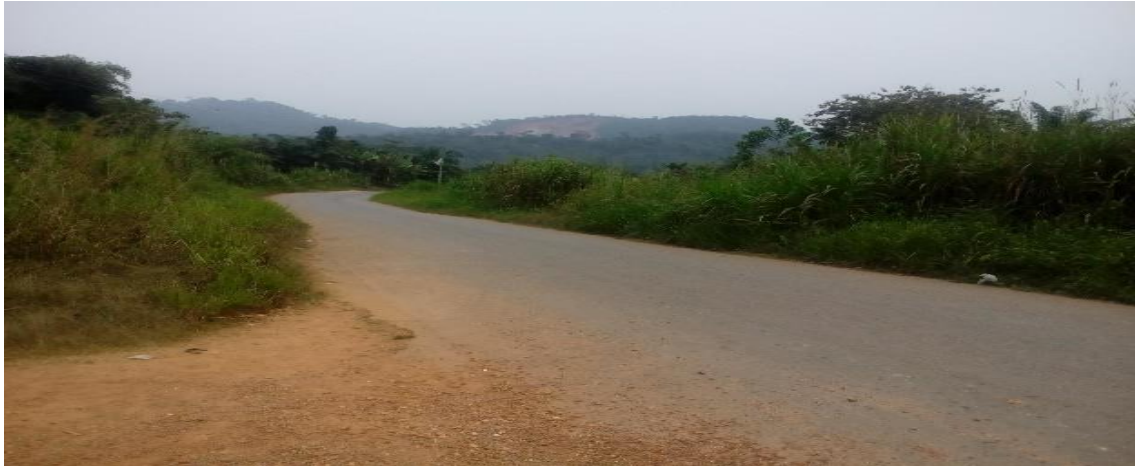
Figure 6.1 Road provided by AGA, Sanso (1)
