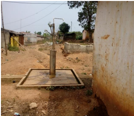
Figure 6.9: Functional borehole, Kokotiasua
