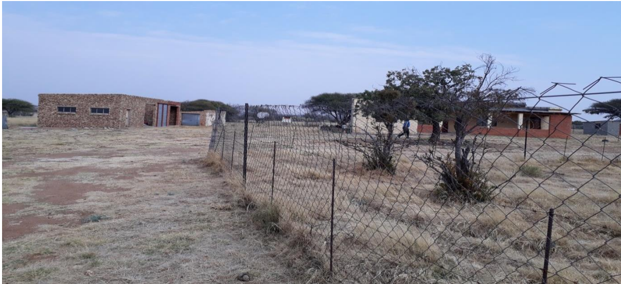
Figure 5.15: Full view of building structures on the Trust's land
