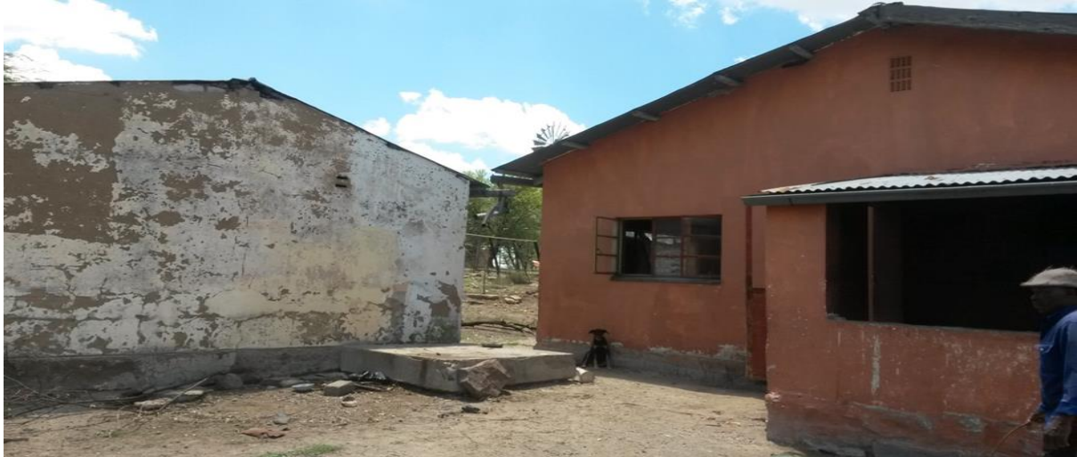
Figure 5.10: Dilapidated farm dwellings on the CPA's land
