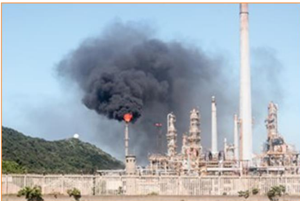
Figure 5.1: Aging refineries in SA requiring upgrade (Oirere, 2017)
