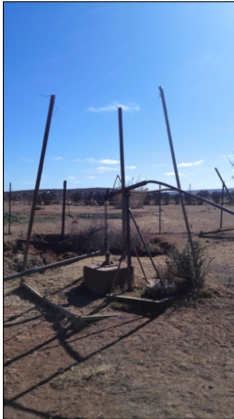
Figure 31: Borehole with Water Pump
