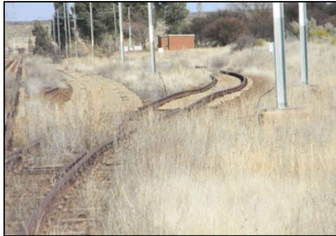
Figure 53: Groenwater Location station, railway tracks
