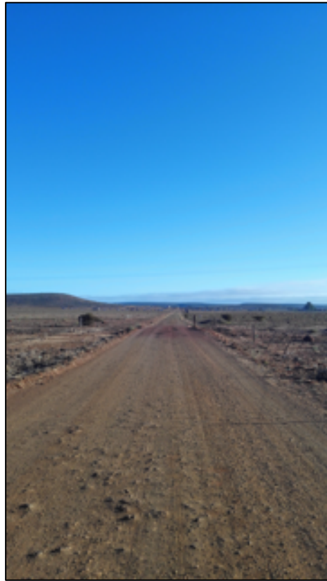
Figure 20: Gravel Road towards Groenwater Location Settlement
