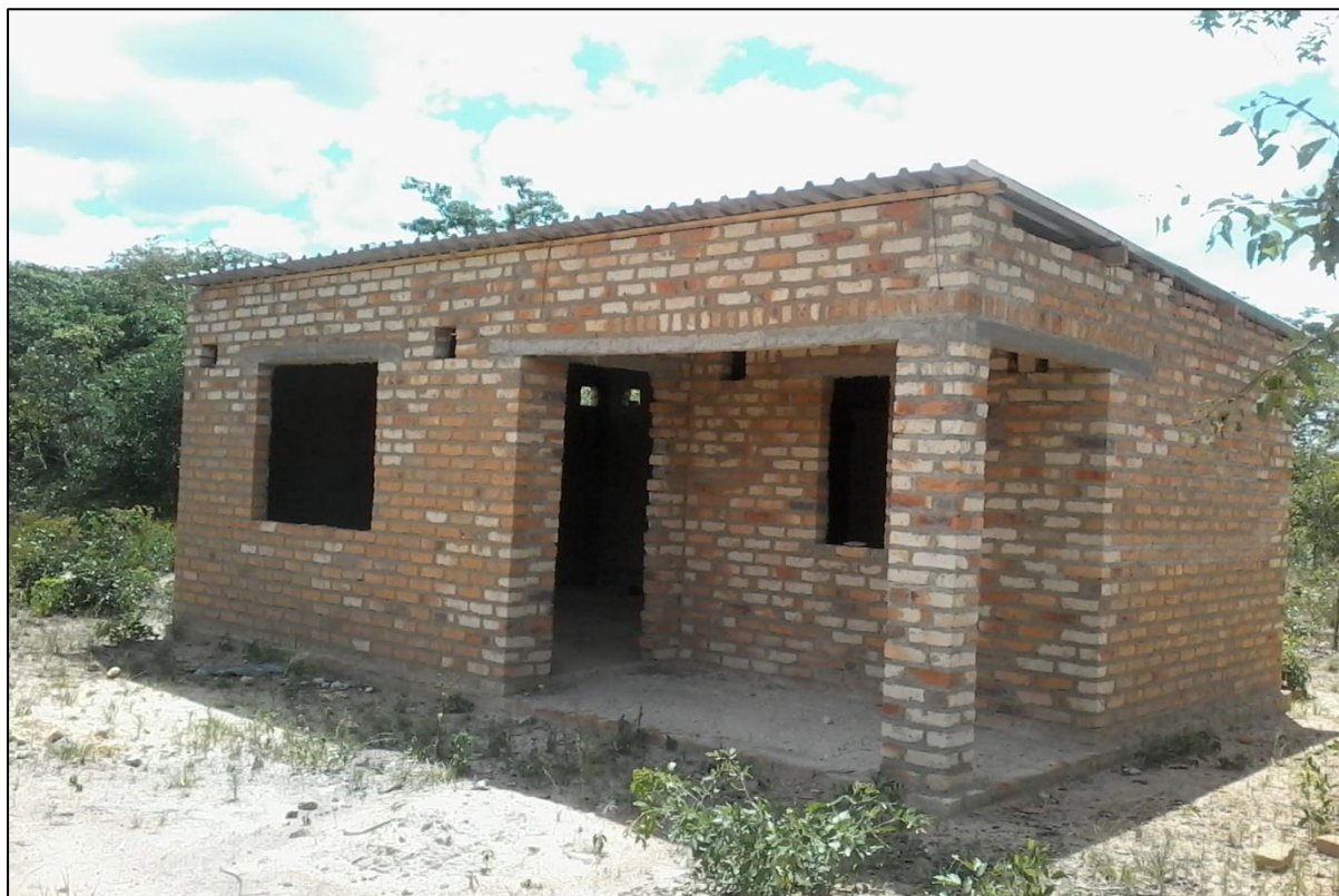
Picture 7.4: A house being built by Mbuya Chirisa's son
