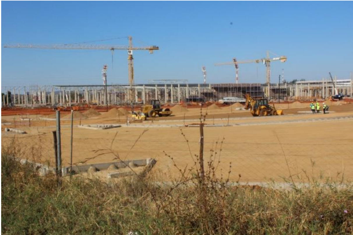
Figure 4.11a: Vegetation cover is removed during construction. (Source: Own).
