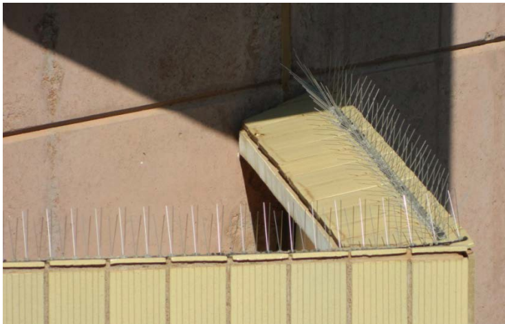
Figure 35: Bird spikes on Cas van Vuuren building of the University of South Africa's Muckleneuk campus
