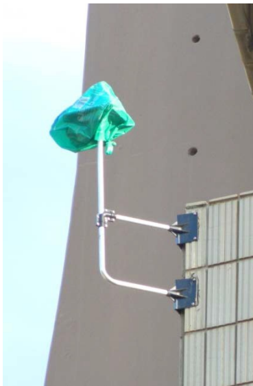
Figure 43: Eagle Eye™ unit covered with a plastic bag by a member of staff to prevent the unit from reflecting light on Theo van Wijk building at the University of South Africa' Muckleneuk campus
