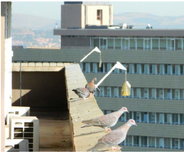
Figure 34: Fire Flags on OR Tambo building of the University of South Africa's Muckleneuk campus
