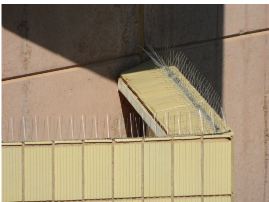
Figure 15: Bird spikes evaluated as a pigeon deterrent on the University of South Africa's Muckleneuk campus
