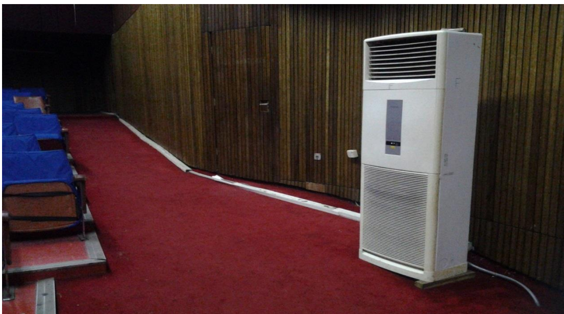
Fig. 12: Church auditorium wall covered with wooden material
