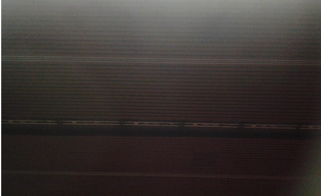
Figure 13: Ceiling of a Church auditorium
