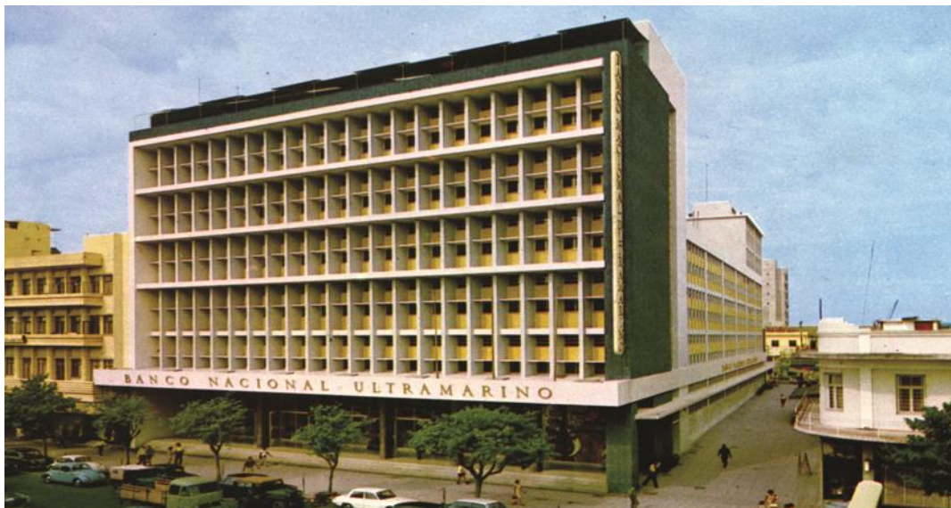
Image of Banco Nacional Ultramarino. Source::Banco de Moçambique Photo collection
