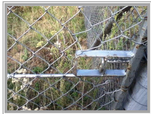
Figure 4.23 & 4.24: Wetland area on school grounds - Good, strong fencing, but no locking mechanism
