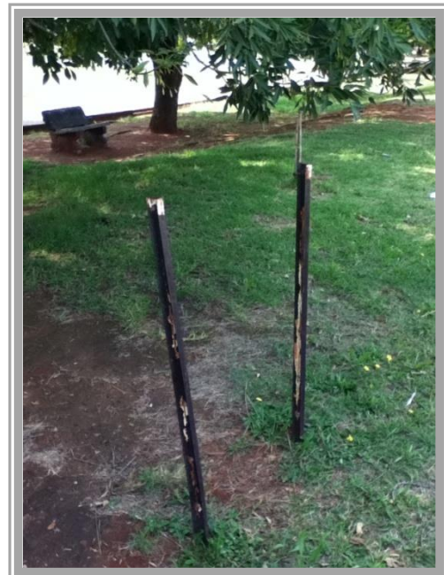
Figure 4.16: Poles of an old gate - a physical hazards posing a risk on a school ground
