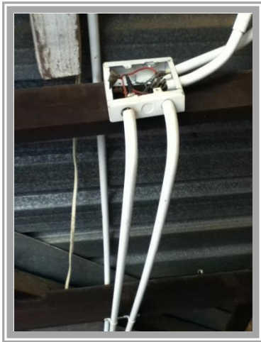
Figure 4.32 & 4.33: Lack of electrical maintenance and safety risk found in the school buildings and on the school grounds
