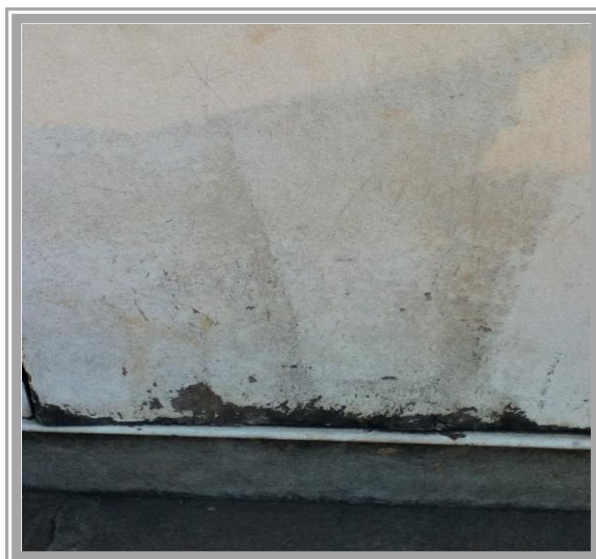
Figure 4.19: Water damage to classroom - poses not only physical risk, but also a biological risk of mould forming school grounds
