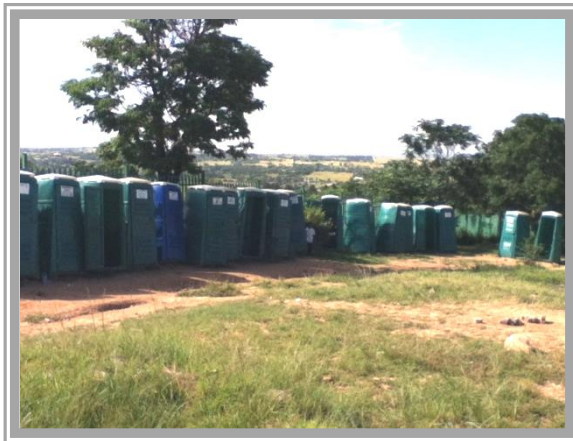
Figure 4.5: Inadequate sanitary facilities - Posing health risk and biological risk
