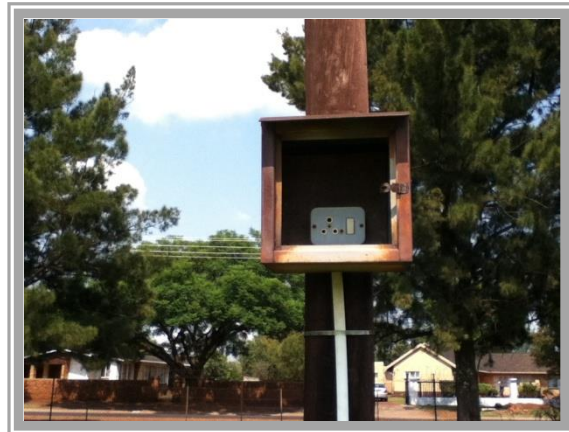
Figure 4.32 & 4.33: Lack of electrical maintenance and safety risk found in the school buildings and on the school grounds
