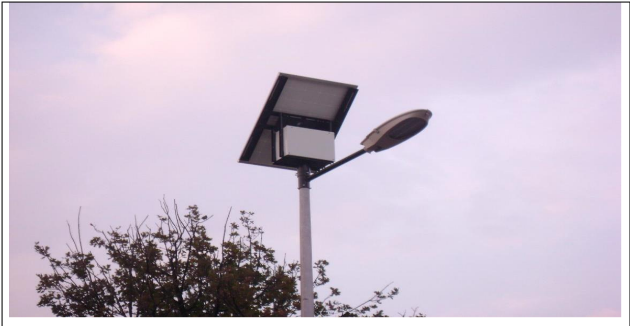
Figure 4.4: Solar powered streetlight in Ekurhuleni
