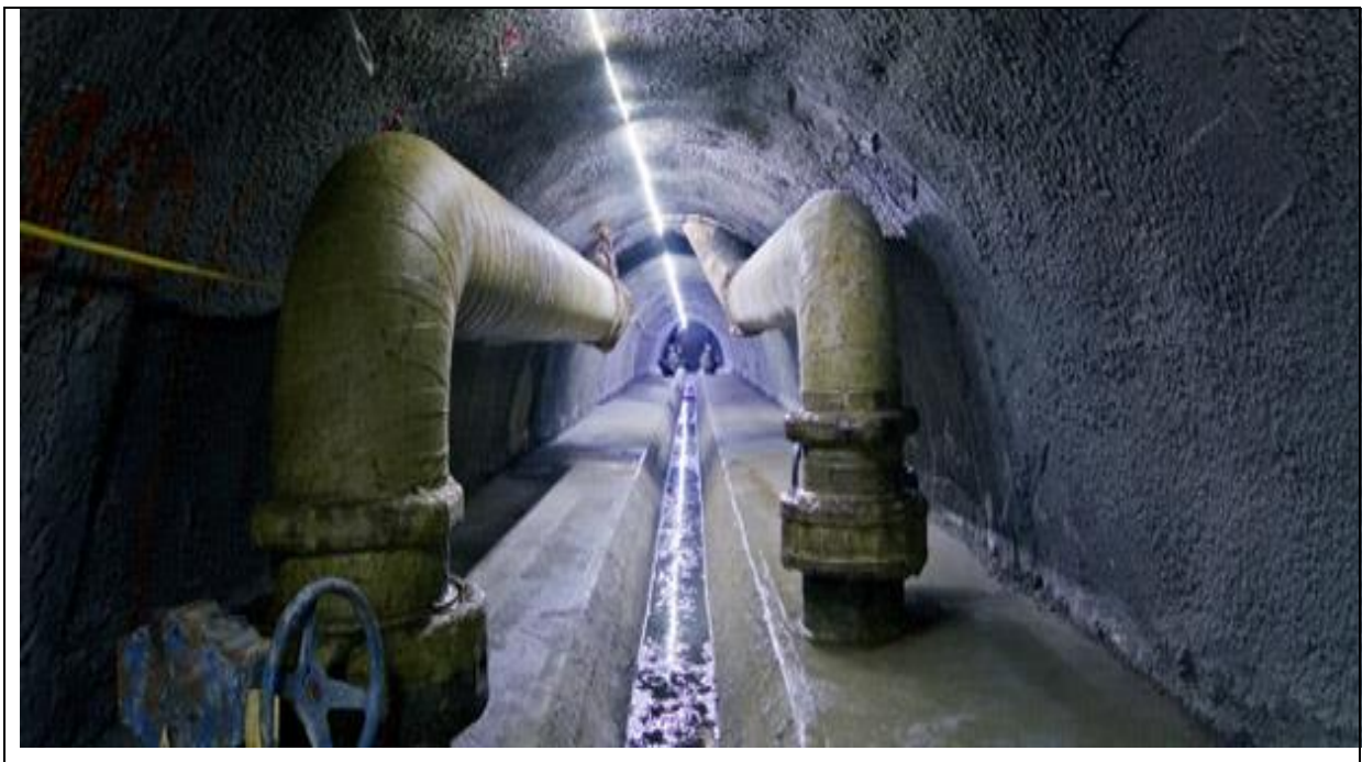
Figure 2.3: Lake Water air conditioning system
