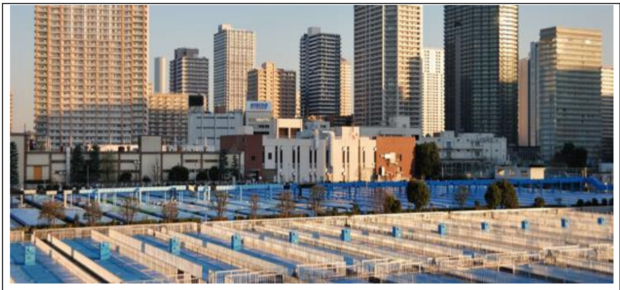
Figure 2.4: Wastewater treatment plant in Tokyo
