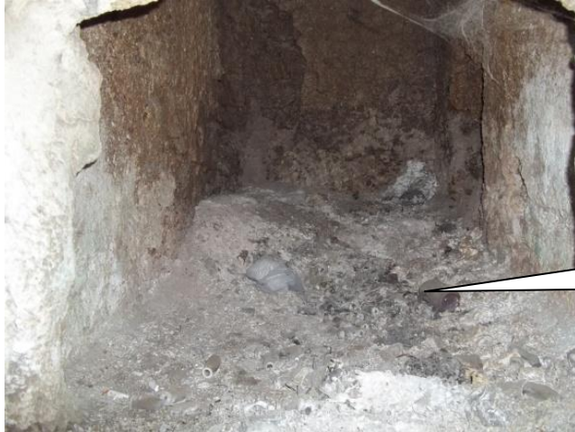
Plate 4.22: Ash residues mixed with tins and bottles at Princess Marina Hospital closed incinerator
