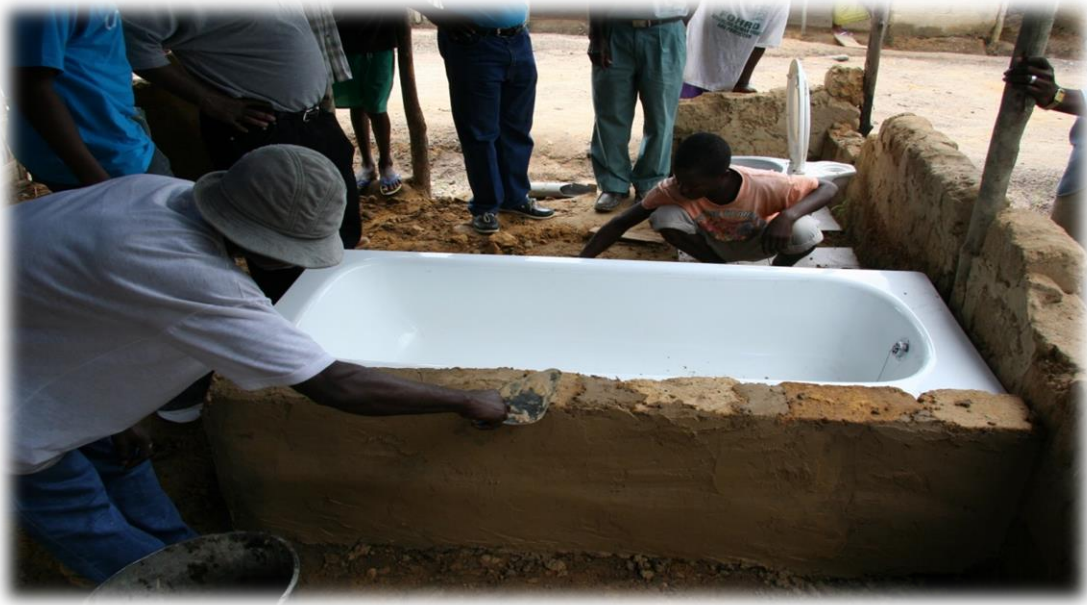
AGHRA APPRENTICESHIP SKILLS TRAINING- PLUMBING
