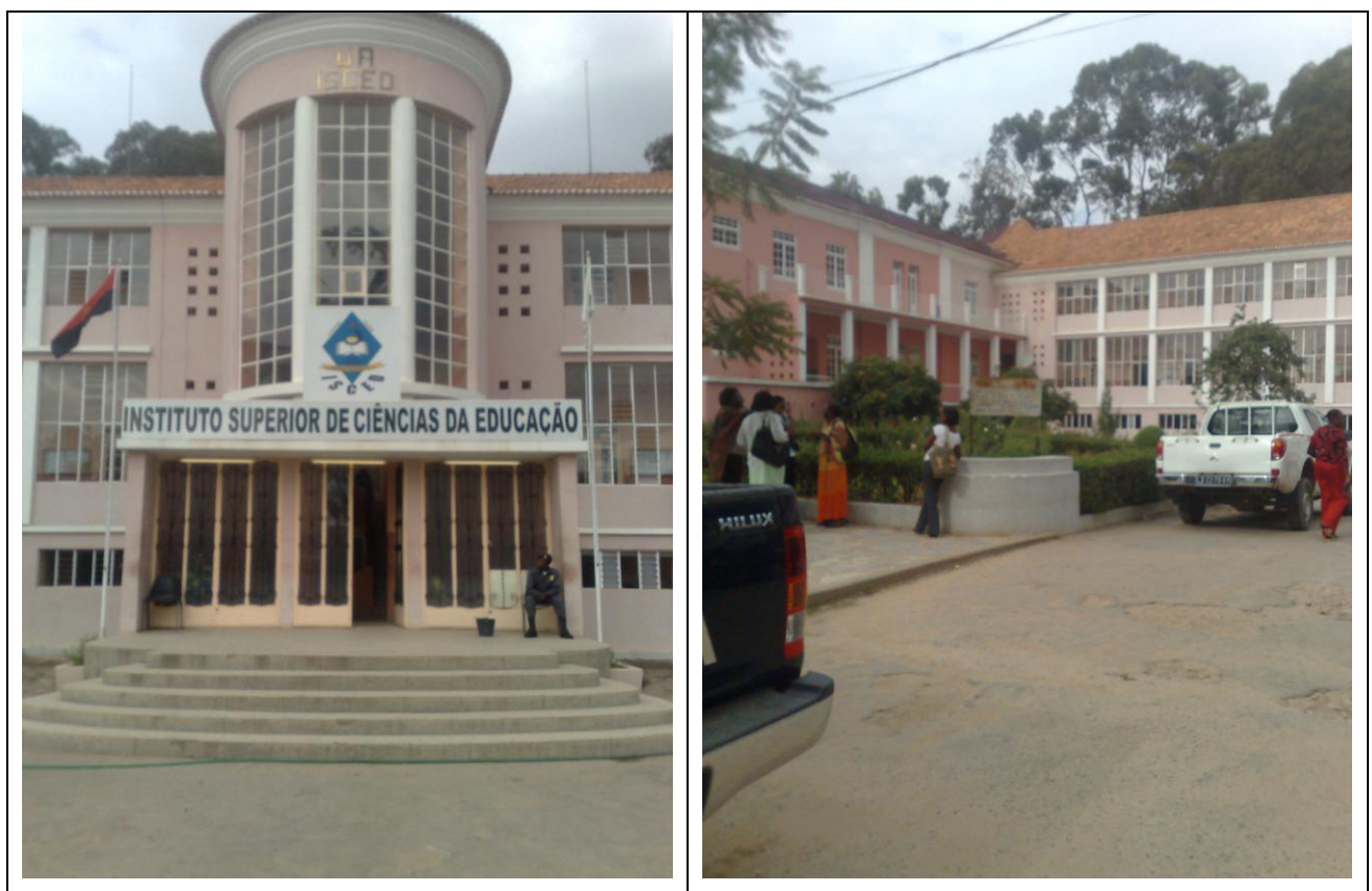
Figure 1.4: The ISCED-Huíla main building
