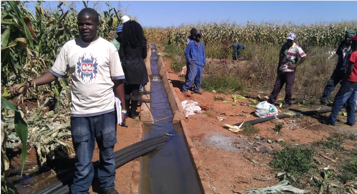
Figure 5.1 Irrigation Expansion underway
