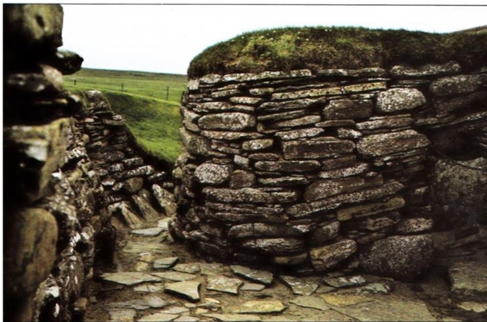
Figure 2-1: Detail of a layered stone wall of a house and flagstone walkway from Skara Brae, Orkney Islands (Wernick 1974:99).
