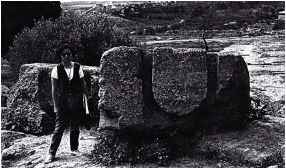
Figure 3-41: A method devised by the Greeks for hoisting consisted of cutting a U-shaped open groove at both ends of a block, through which ropes could be threaded (Phoca & Valavanis 1999: 110; Ressler 2014:27).
