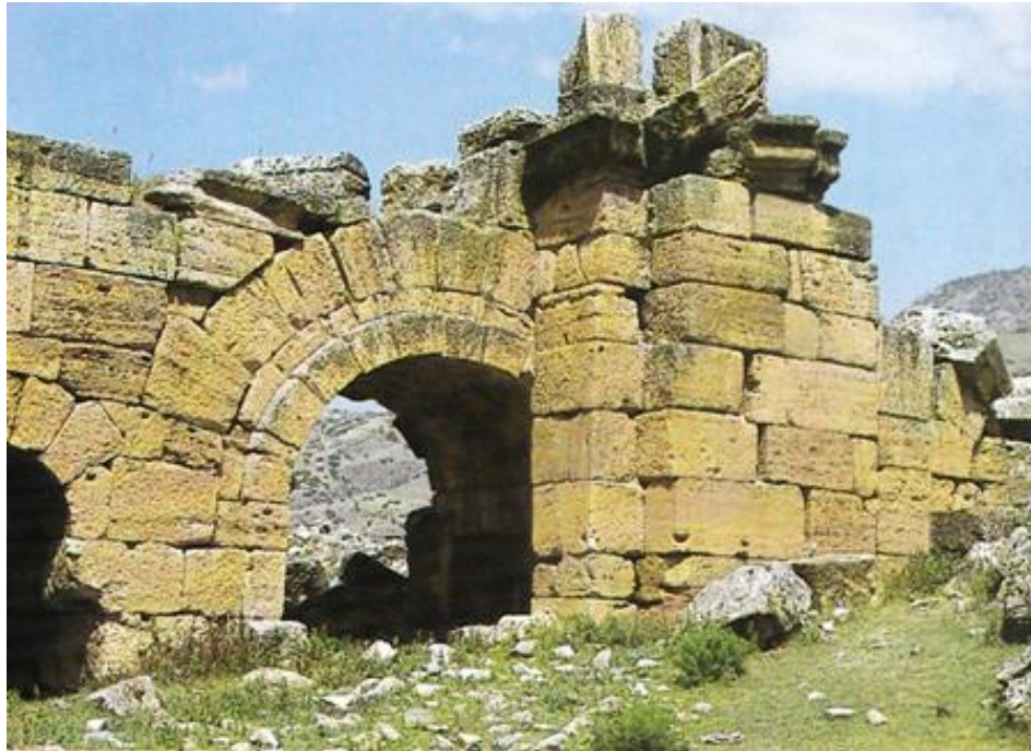
Figure 2-5: White travertine from Pamukkale, has changed colour due to exposure to air (Kekeç 1997:41).
