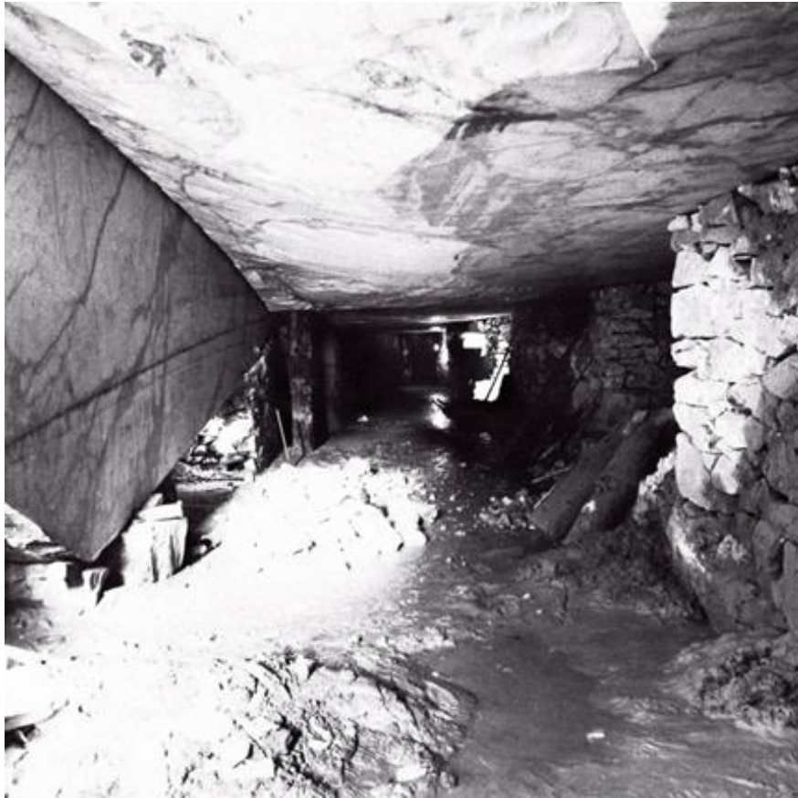
Figure 3-6: Interior of a gallery type quarry. Note the stacked stone pillars on the right (Mannoni 1985:92).
