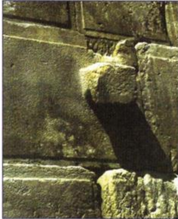
Figure 3-42: Small stone protrusion on a block of stone left by the stonemason to enable hoisting of the block (Ritmeyer 2006:134).
