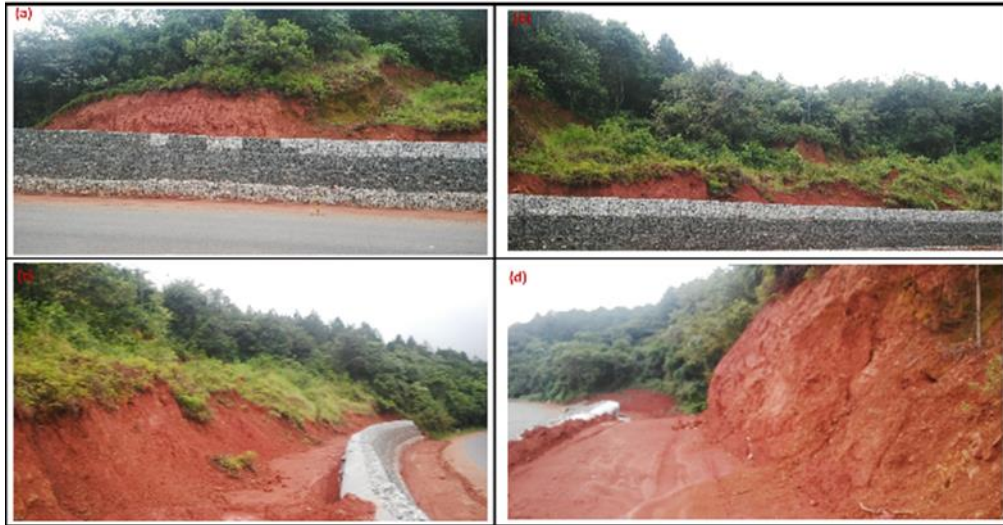
Figure 4.3 Occurrences of post landslides along the R523 road
