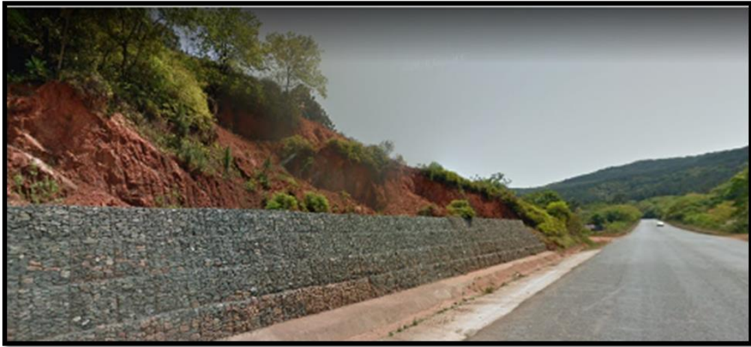
Figure 4.4 The effective gabion walls along R523 road
